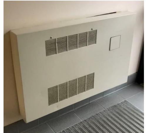
Figure 11: CUH-4, Hydronic Cabinet Heater
