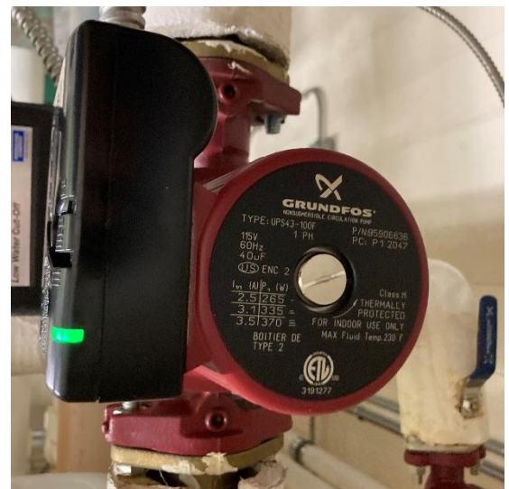
Figure 9: Grundfos Inline Three Speed Boiler Pump
