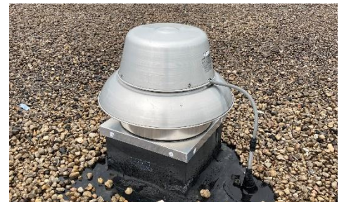
Figure 3: Jenco Downblast Exhaust Fan
