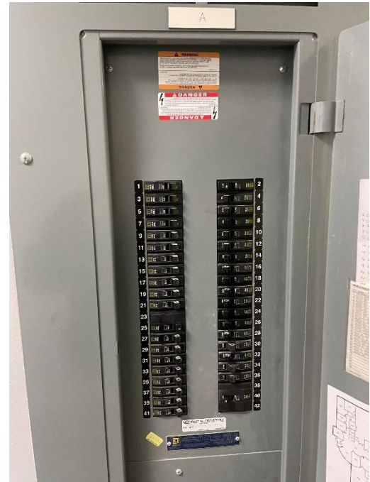
Figure 25: Panelboard Interior
