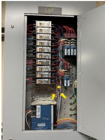
Figure 19: Existing Lighting Contractor
