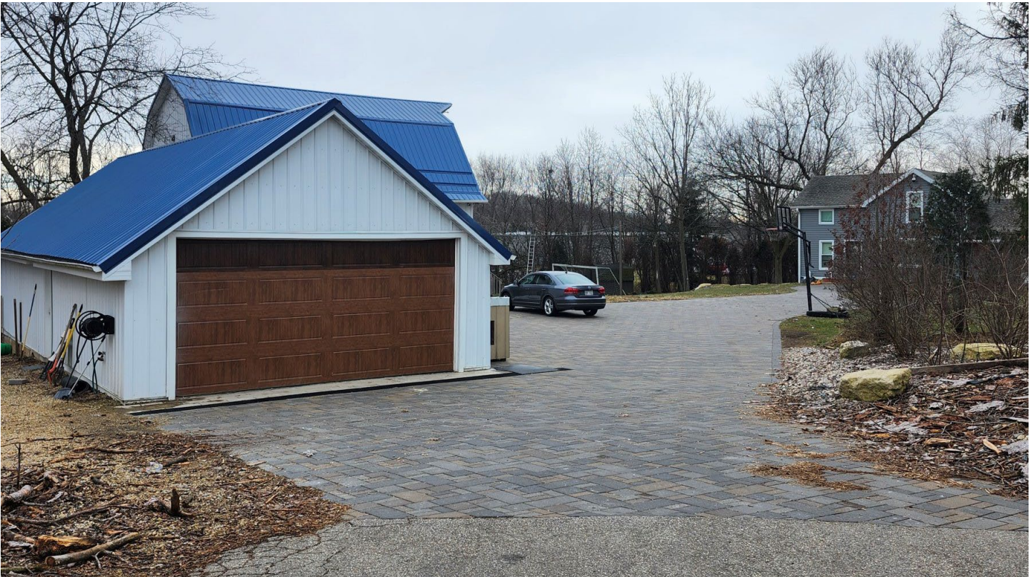
Photo 1: From shared driveway facing southwest
