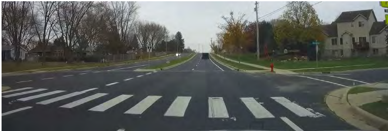
Siggelkow Road, looking east at Black Walnut Drive (note different crosswalk styles and lack of curb ramp detection field)
