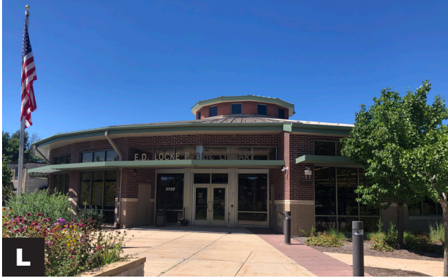
L Building Envelope: The overall condition of the building is in good working order. Insulation appears adequate, brick appears in good shape and there were no large indications of water infiltration.
