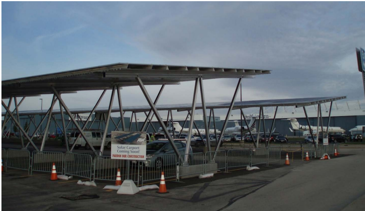
Figure 13- Example solar carport in Wisconsin
