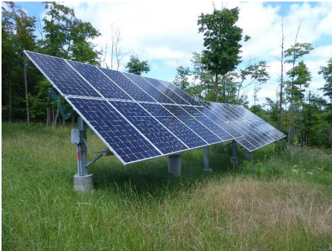
Figure 7- Example of ground mounted solar PV system
