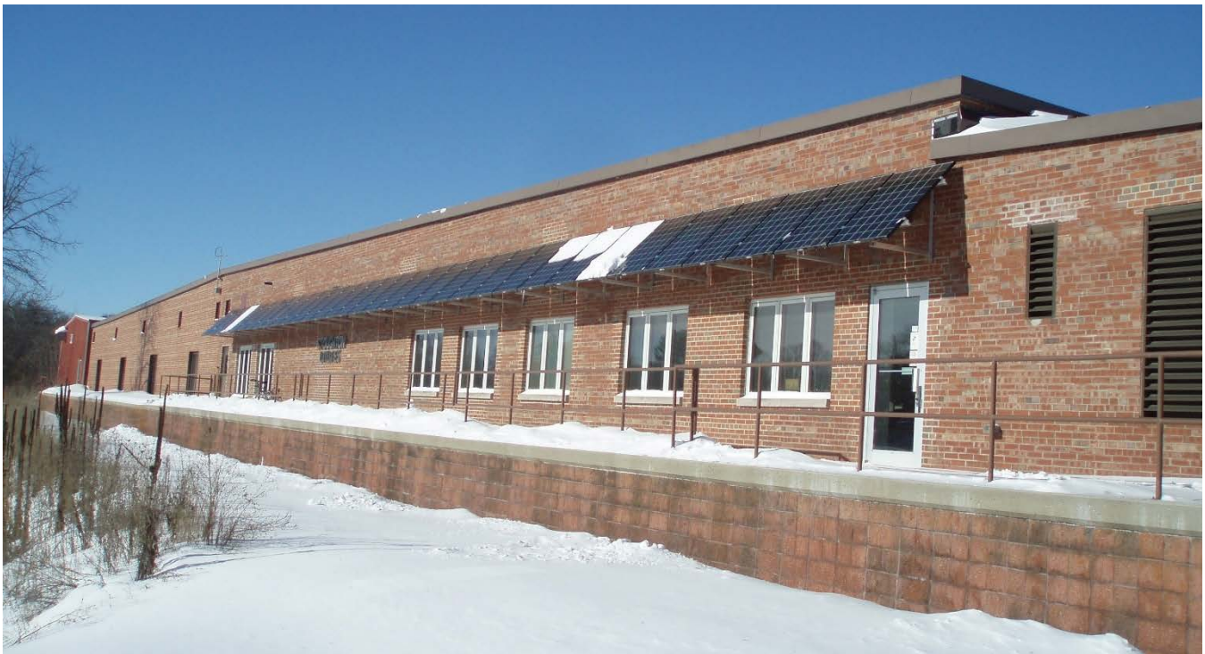
Figure 8- Example of south-facing exterior wall mounted panels
