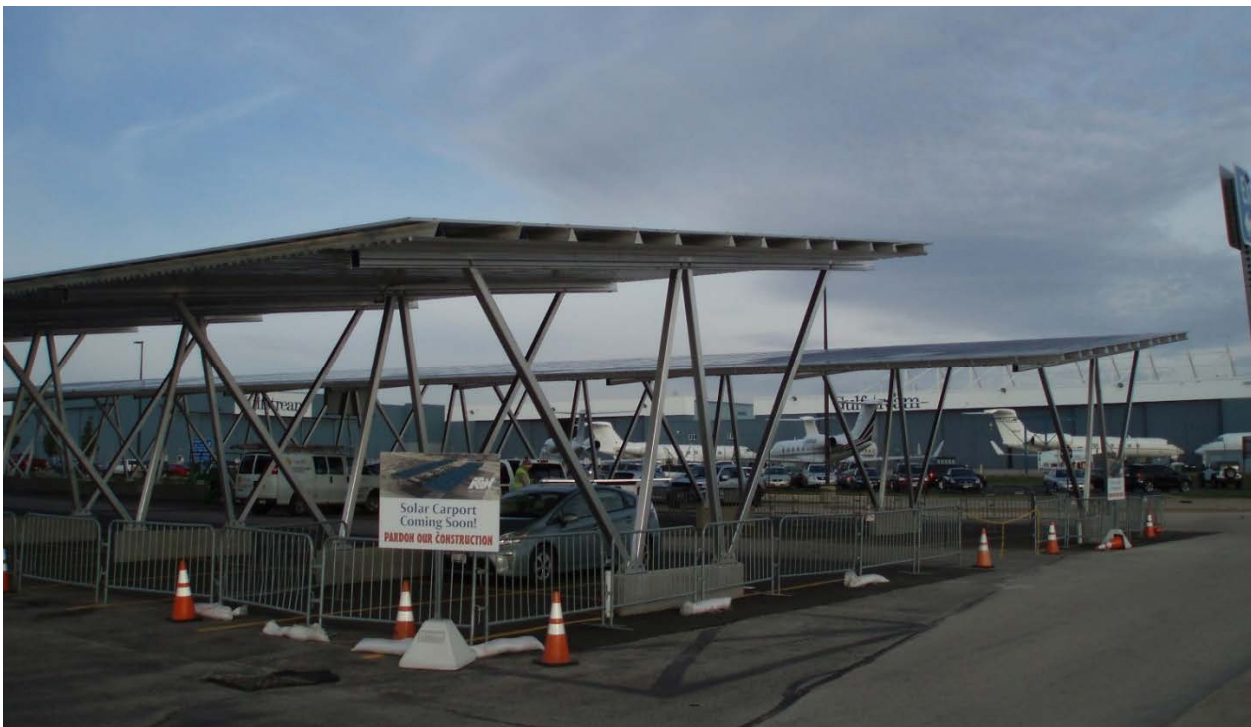
Figure 13- Example solar carport in Wisconsin
