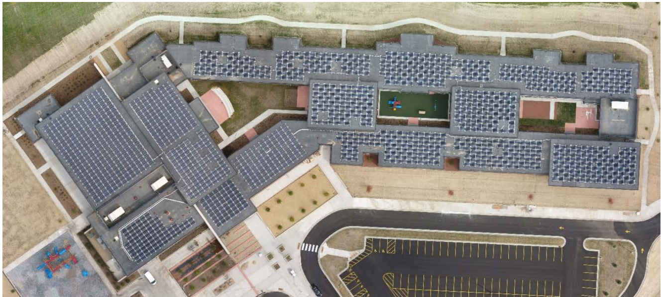
Figure 5- Example solar PV installation at Oregon Forest Edge Elementary School - a similar PV system is proposed for the new PSB project
