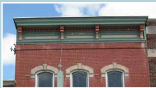
FLAT ROOF W/ CORNICE
