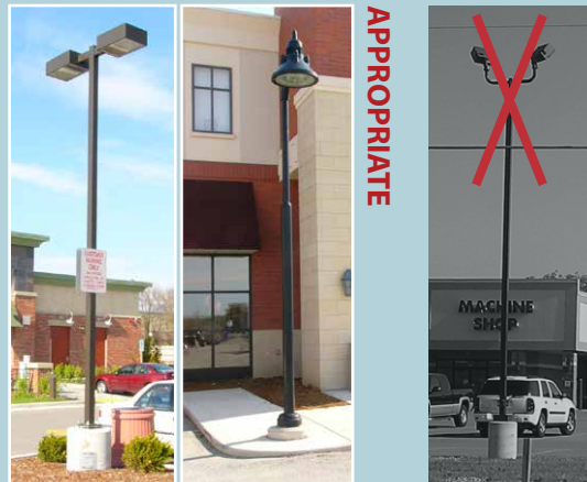
The two images on the left show good examples of low parking lot fixtures that project light only where it is needed, while the far right image shows an excessively tall light that is directed outward, creating glare and light trespass.
