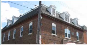
MANSARD ROOF (with dormers)
