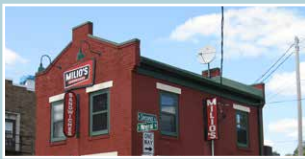
PITCHED ROOF W/ PARAPET
