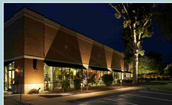
INAPPROPRIATE Above example illustrates excessive lighting leading to light pollution.
