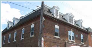
MANSARD ROOF (with dormers)
