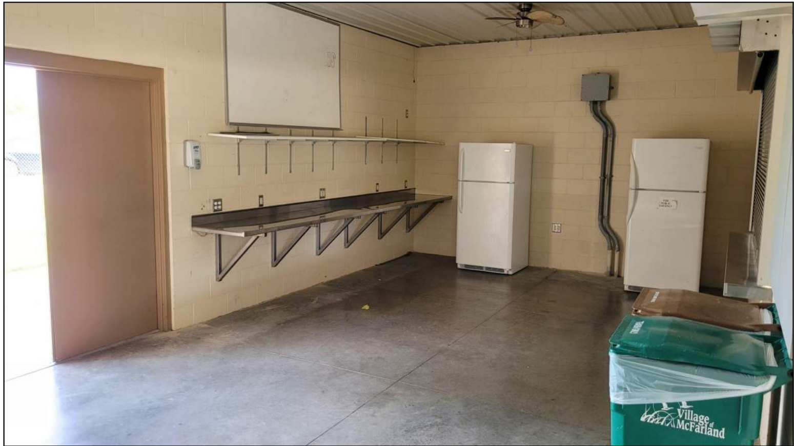
EXISTING CONCESSIONS WALL - NORTH
