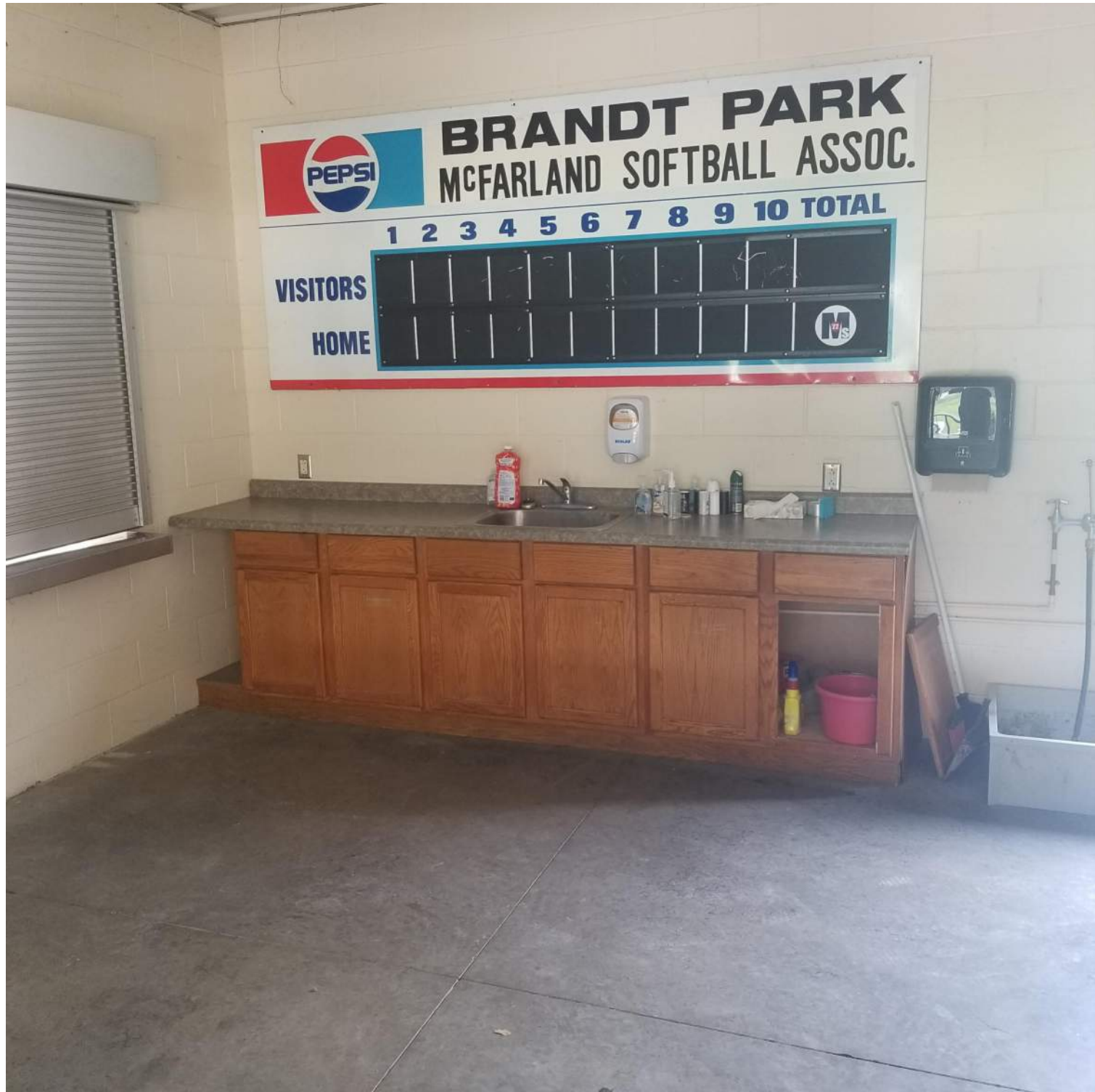
EXISTING CONCESSIONS WALL - SOUTH
