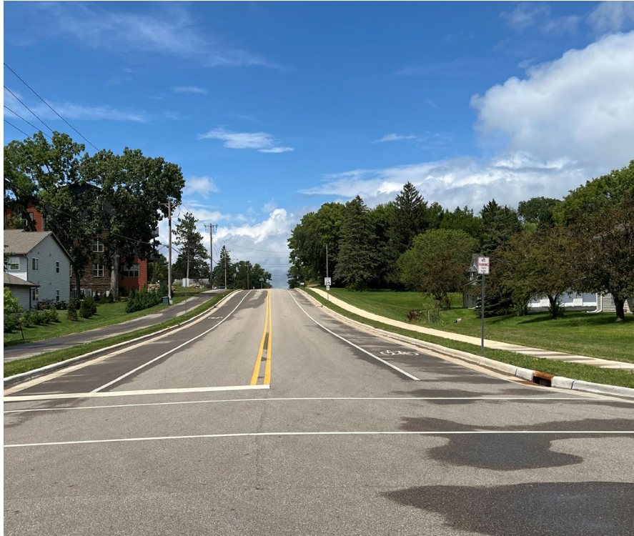
Terminal Drive road, utility, bike lanes, off-road path, and sidewalk infrastructure
