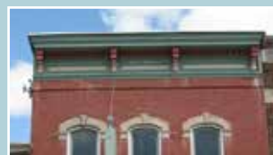
FLAT ROOF W/ CORNICE
