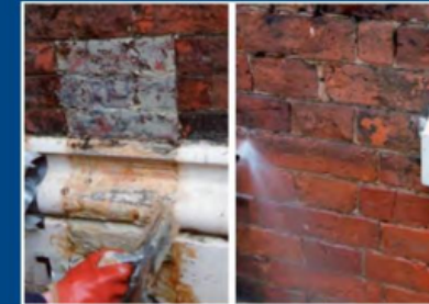
ALLOWED Chemical / Softblast Cleaning
