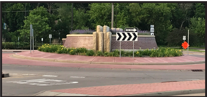
Short retaining wall with stone veneer, McFarland “M” logo and Rhus aromatica (fragrant sumac) or other ground cover plantings less than 30” tall.
