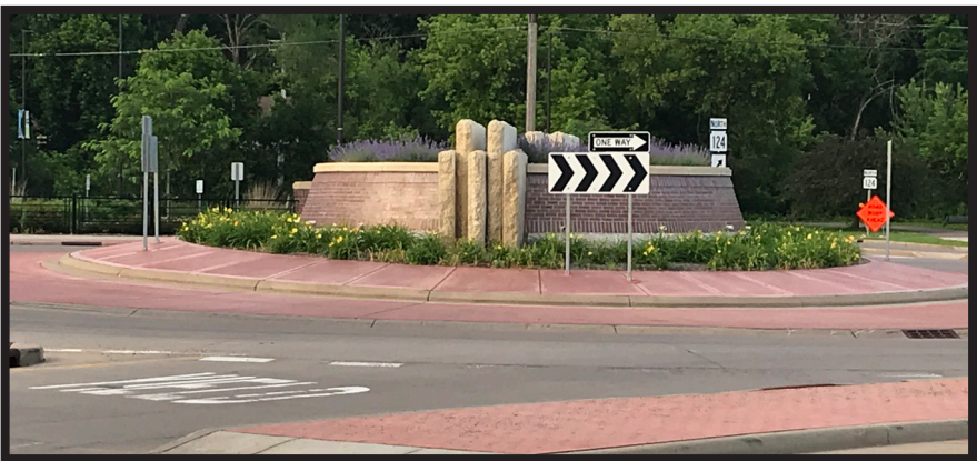
Short retaining wall with stone veneer, McFarland “M” logo and fragrant sumac ( Rhus aromatica ) or other short ground cover plantings.
