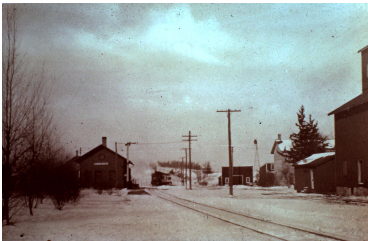
Early 1900 photo looking west. McFarland House center/right behind Eighmy grain elevator.
