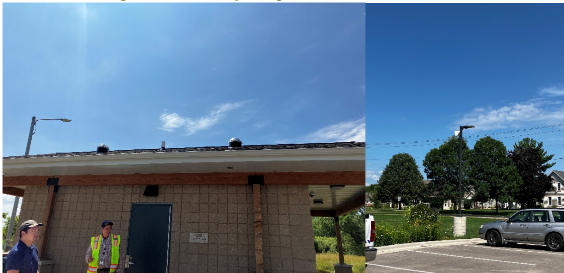
Figure 20: McFarland Dog Park shelter and parking lot
