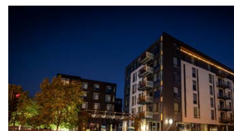
City of Milwaukee North End
