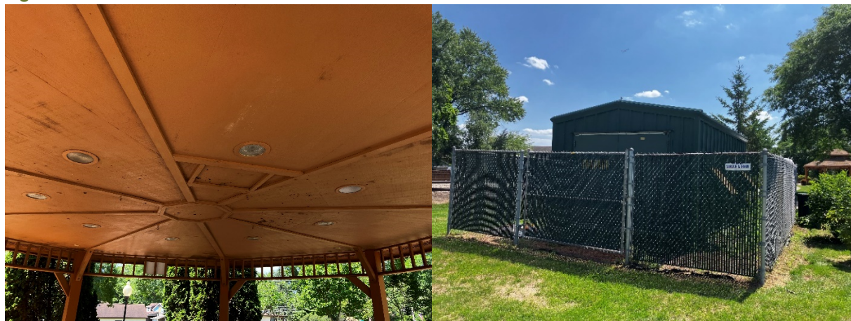
Figure 22: Farwell St Gazebo/ Arnold Larson Park and shed
