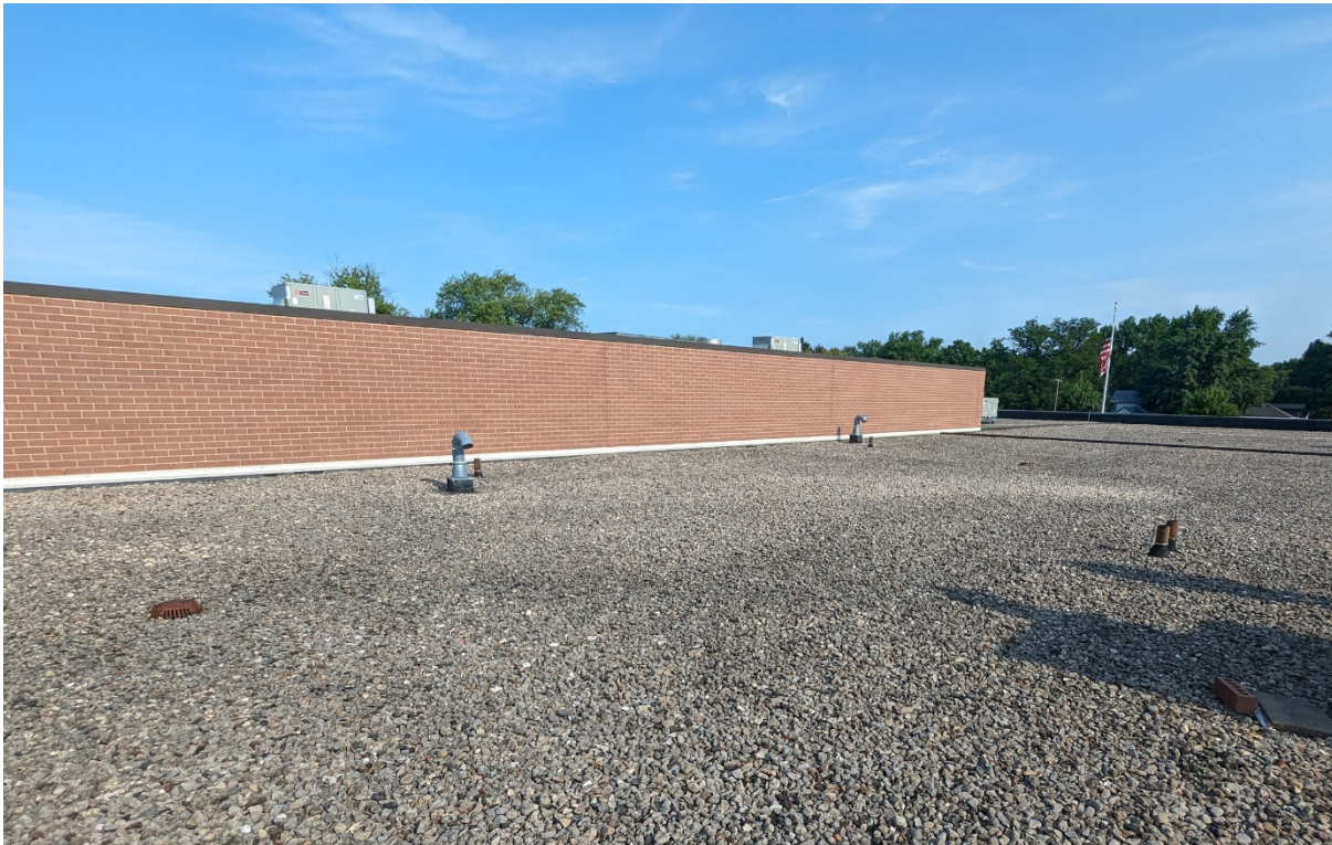
Figure 7 Existing Roof Structure
