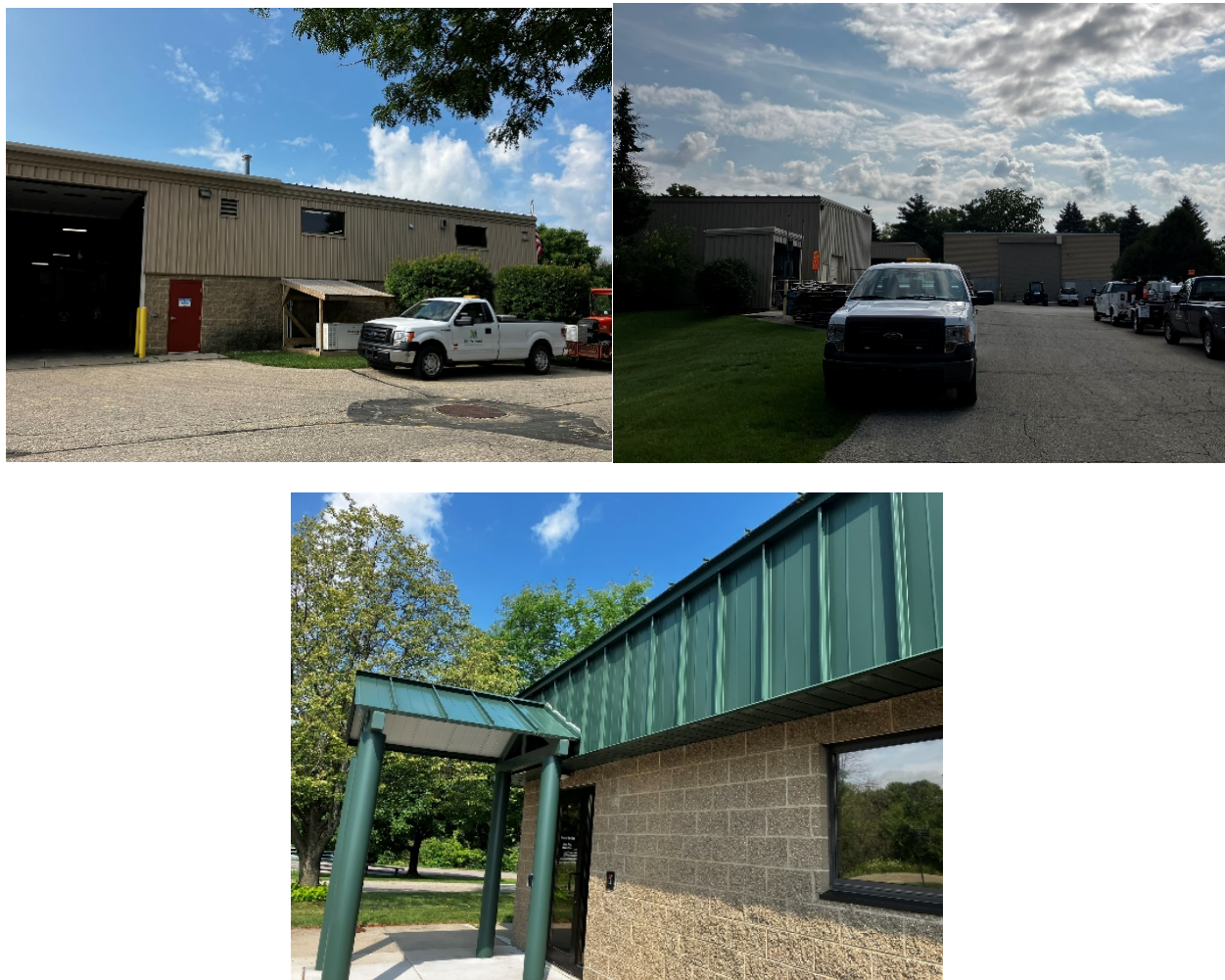
Figure 10: McFarland Public Works Building
