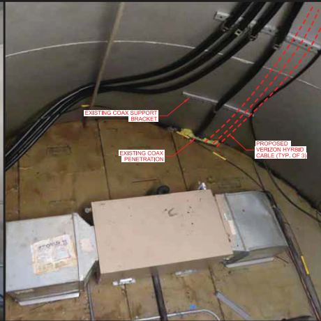
B COAX ROUTING (1ST PLATFORM)
