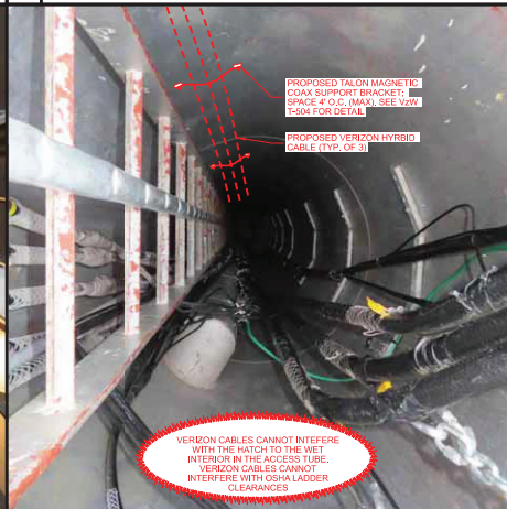
E COAX ROUTING (ACCESS TUBE)
