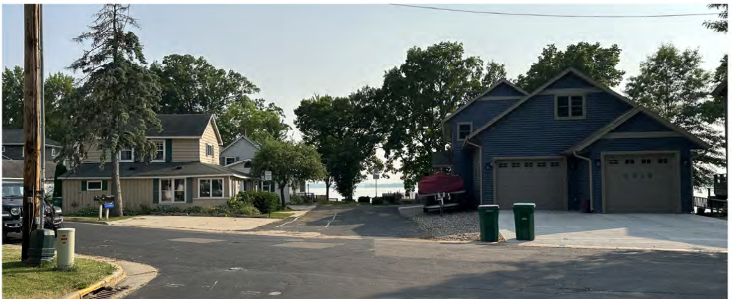
AFTER – 5018 Card Street, McFarland, WI 53558 (on right - directly across the street from the subject property) June 2023
