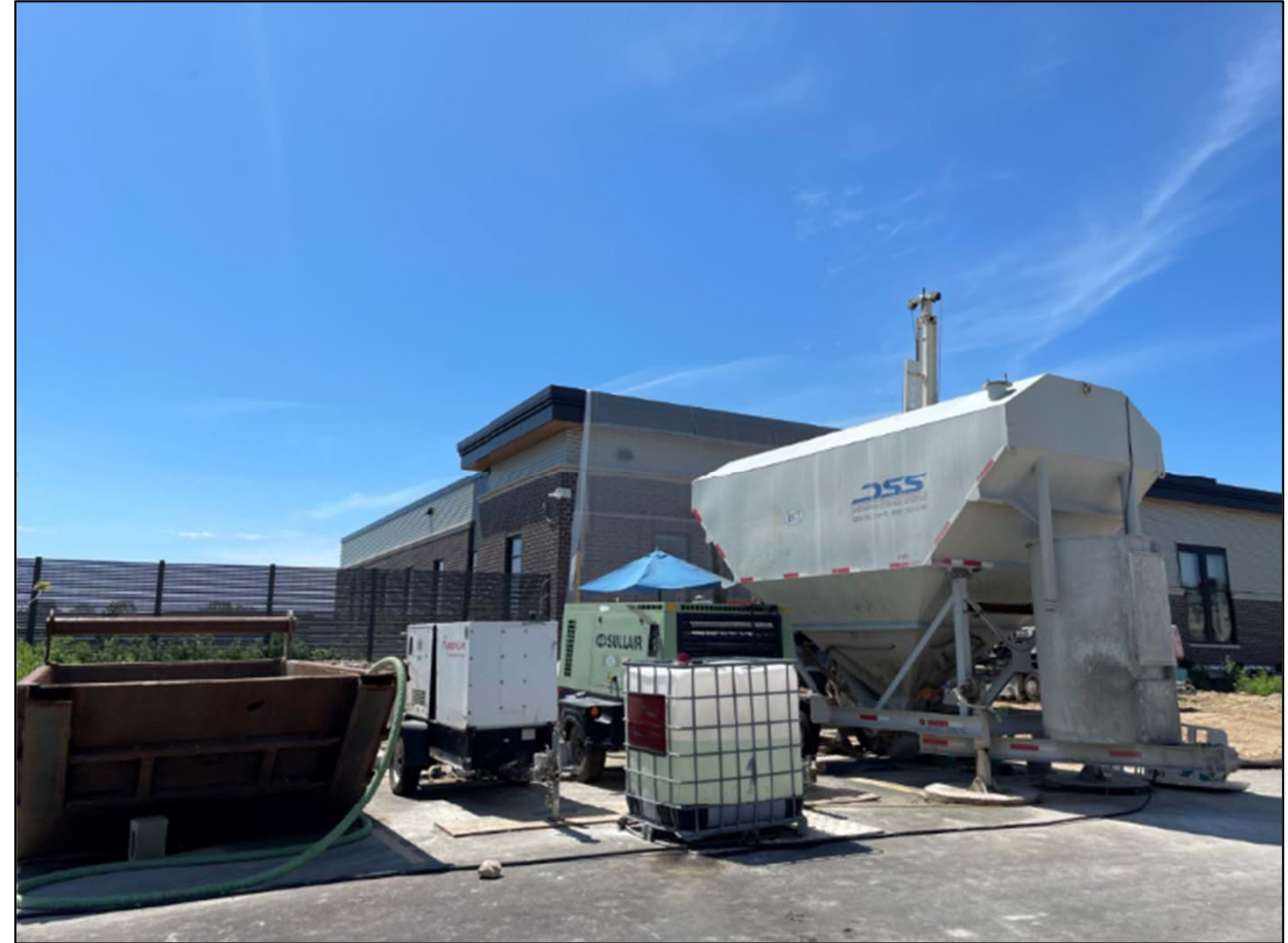
Sinkhole Grouting Operation
