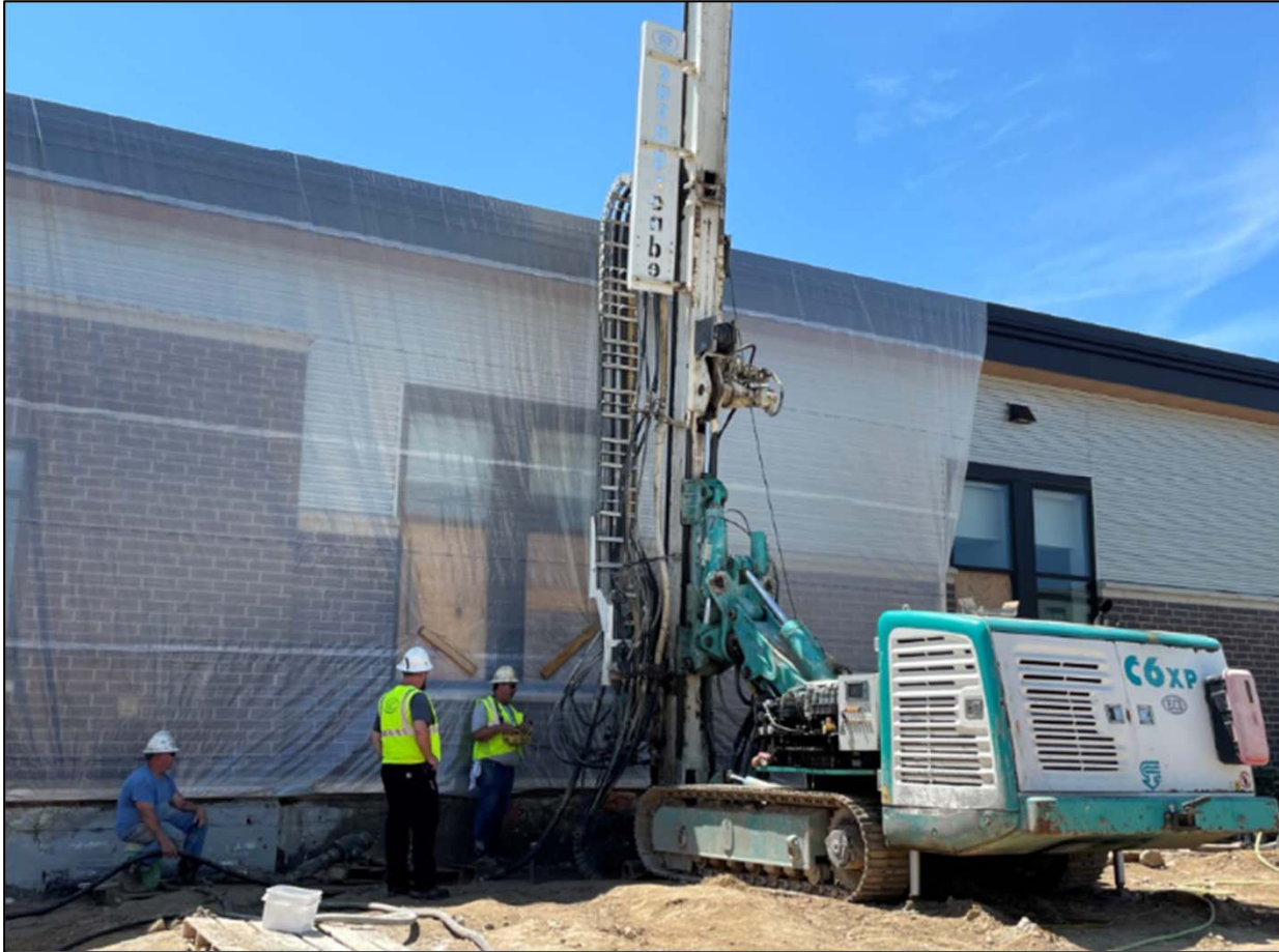
Sinkhole Grouting Operation
