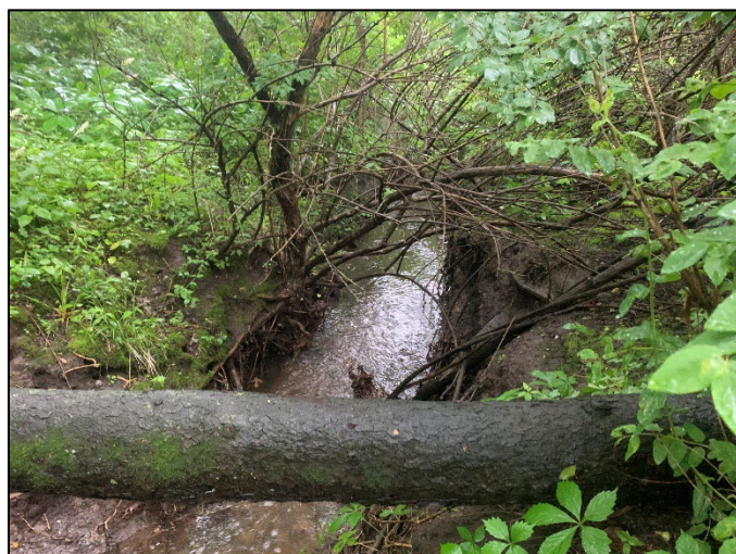
Photo 30. Severe gully erosion downstream of stormwater discharge pipe in Thrun Marsh Conservancy (large precipitation event on June 8, 2022).
