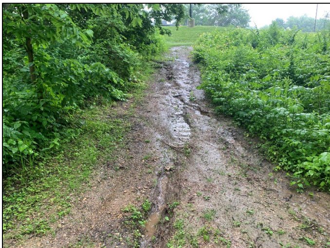
Photo 33. Rill erosion on hiking trail at Indian Mound Conservancy caused by concentrated runoff from the Indian Mound Middle School (large precipitation event on June 8, 2022).
