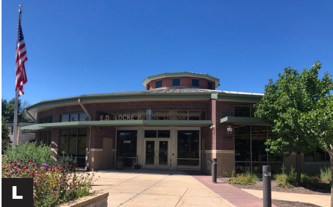
L Building Envelope: The overall condition of the building is in good working order. Insulation appears adequate, brick appears in good shape and there were no large indications of water infiltration.
