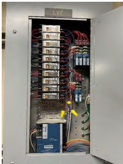
Figure 19: Existing Lighting Contractor
