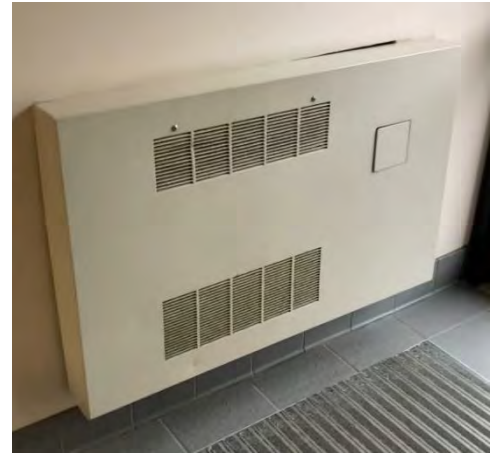
Figure 11: CUH-4, Hydronic Cabinet Heater
