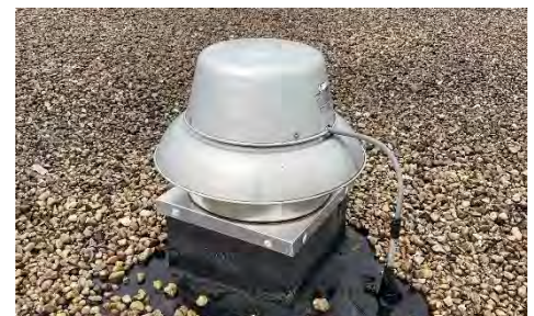
Figure 3: Jenco Downblast Exhaust Fan
