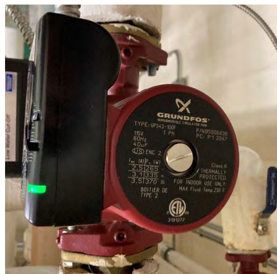
Figure 9: Grundfos Inline Three Speed Boiler Pump
