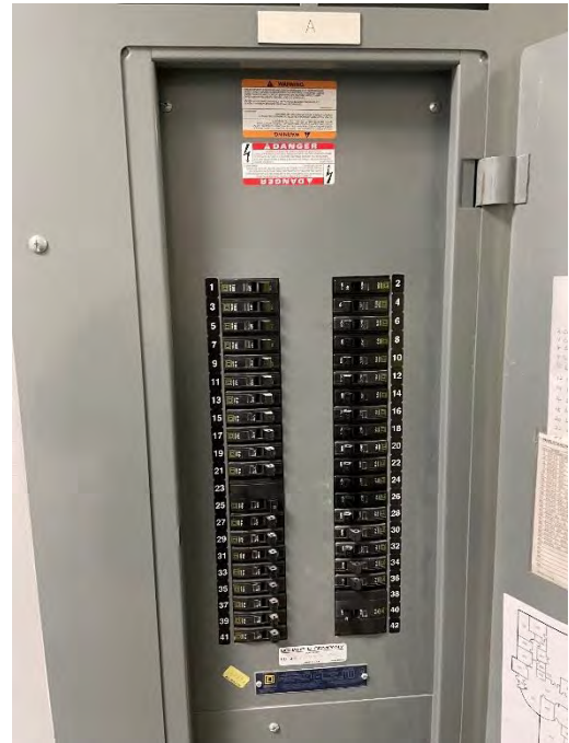
Figure 25: Panelboard Interior
