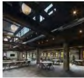
Character of Indoor Space Exposed Ceiling
