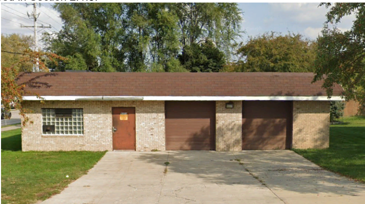
Well 3 Wellhouse Exterior
