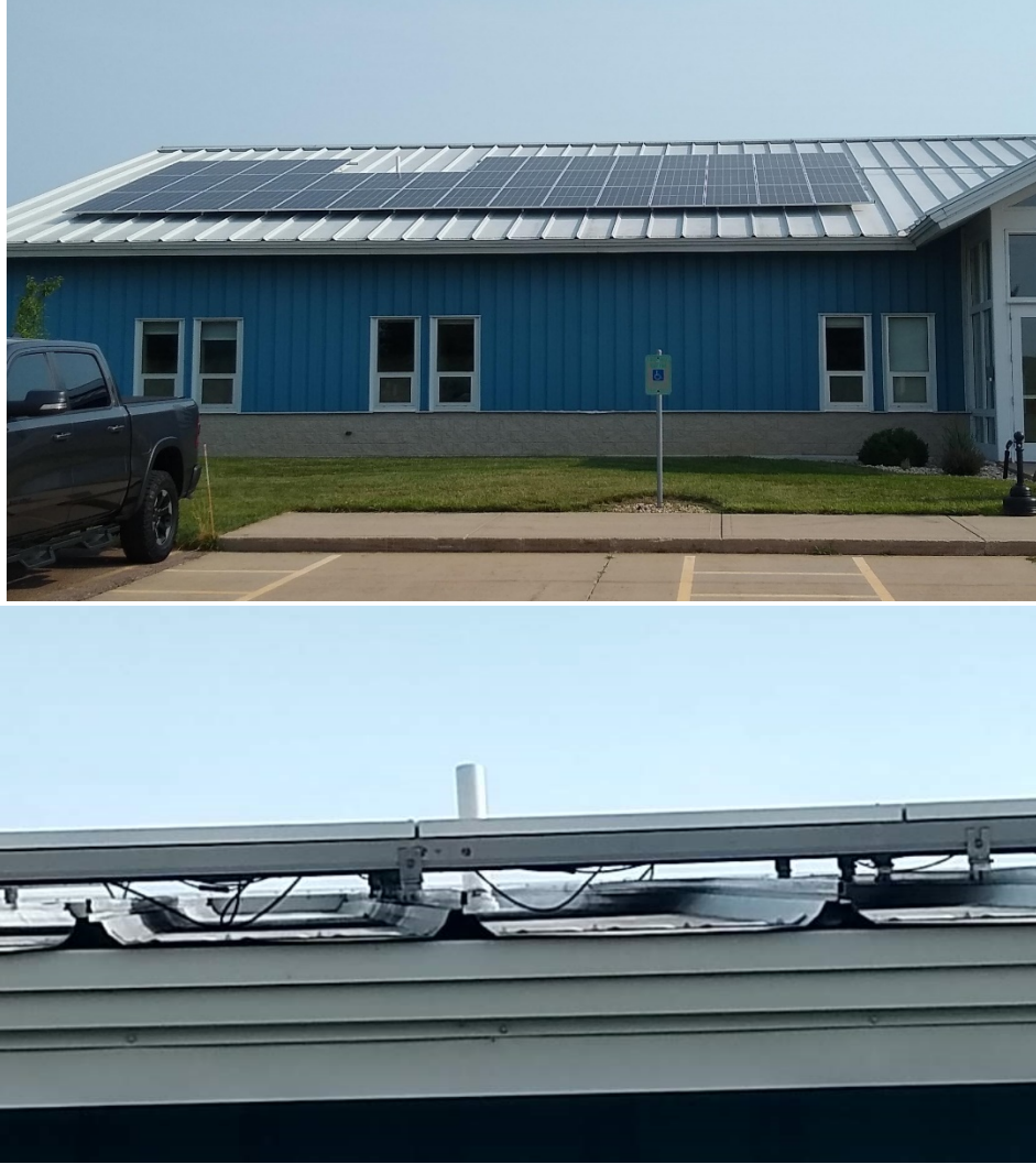
Figure 6- Sample image of flush mount panel racking on standing seam roof
