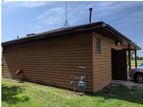
Well 4 Wellhouse Exterior
