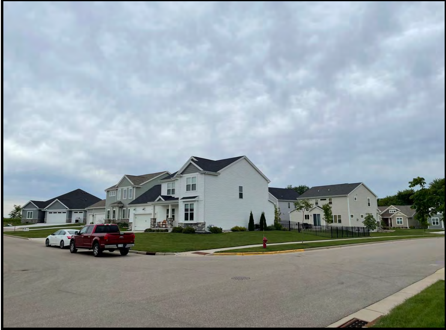
Photo Location Directly West – {After}
