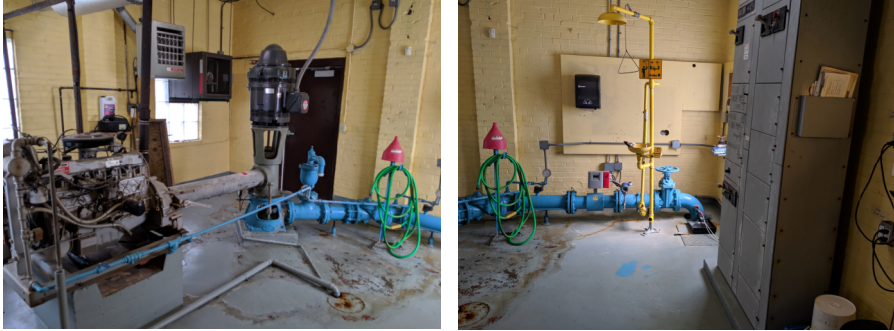
Well 1 Building Interior
