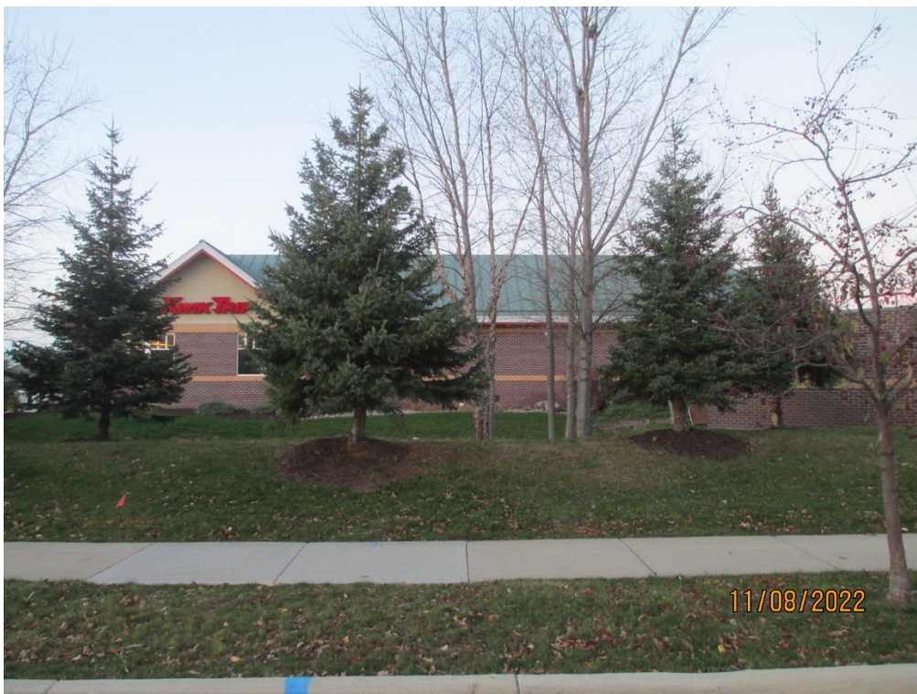
View of rear building from Burma Road.
