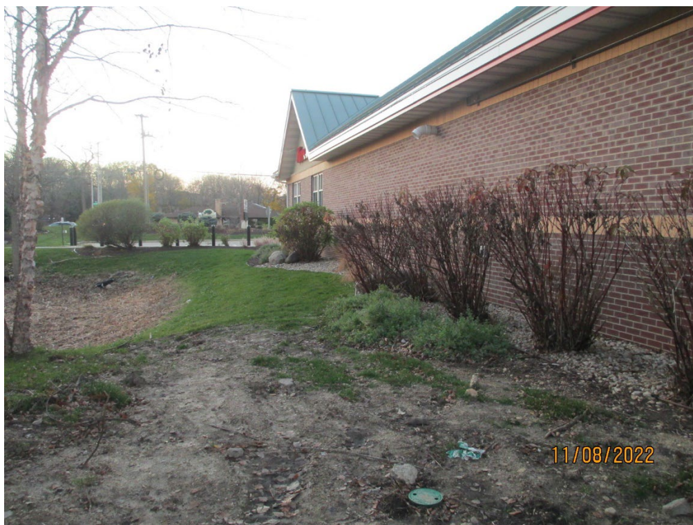
View of rear of building proposed for expansion
