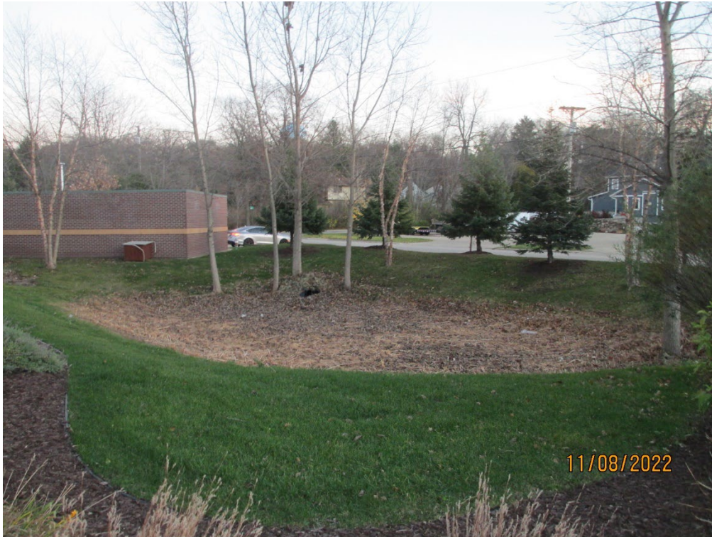
View of rear stormwater basin
