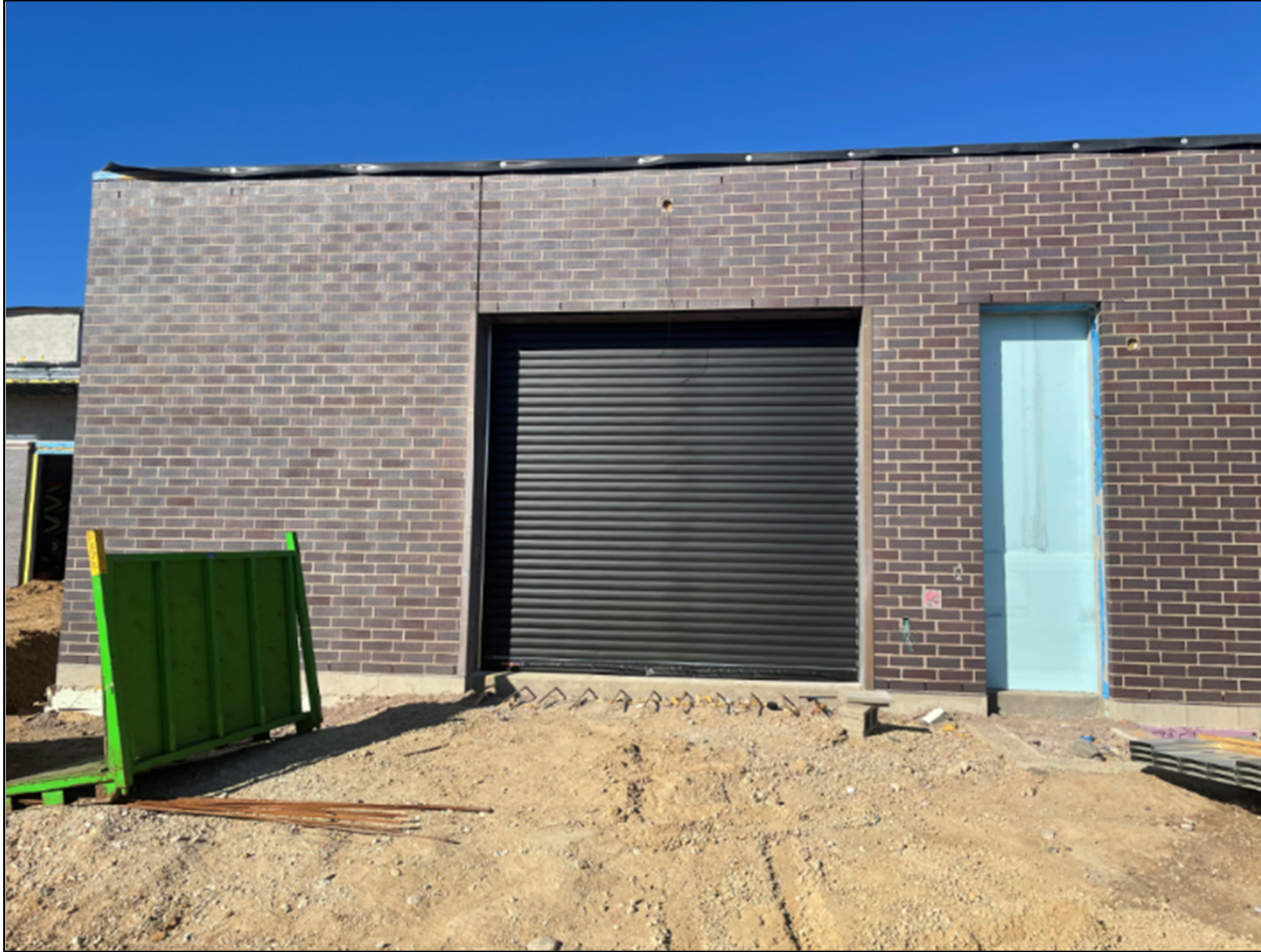
Overhead Door Installed at PD garage
