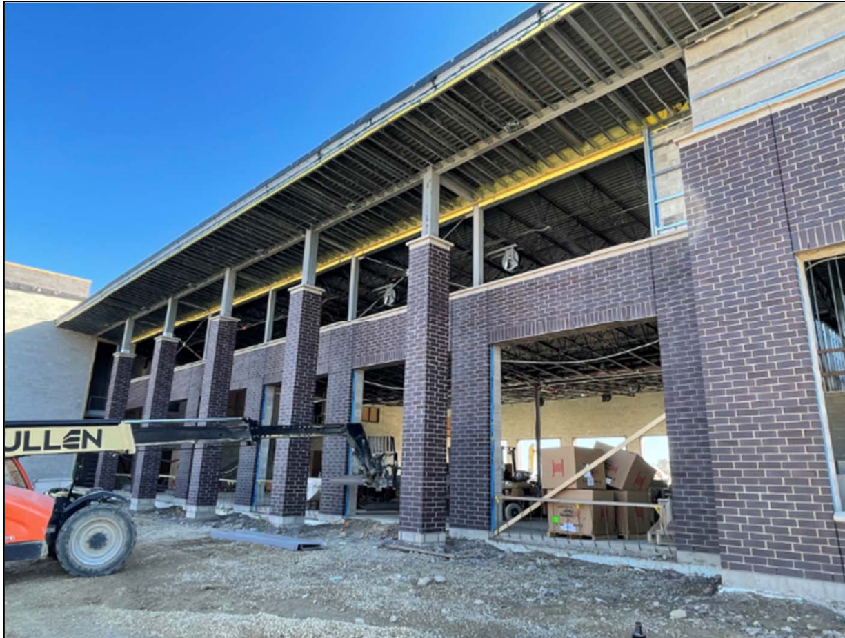
Masonry, Steel and Roof at Fire Department Apparatus Bays
