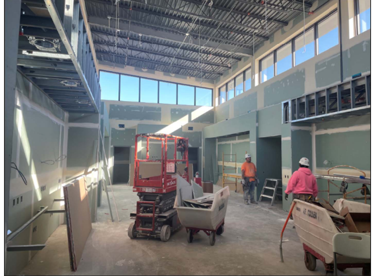
Drywall at the Squad Room
