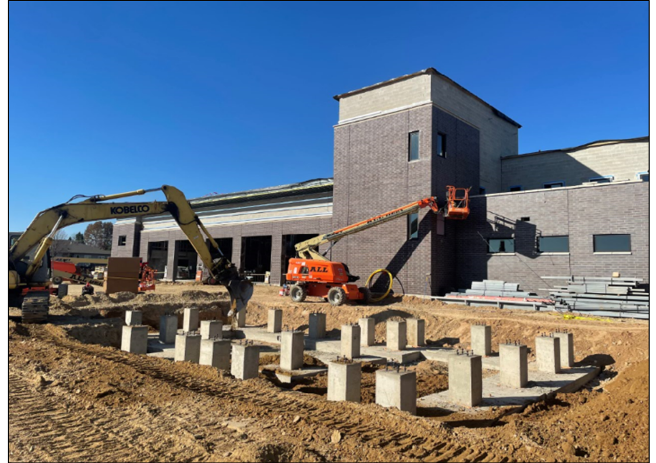
Foundations for Electrical Enclosure
