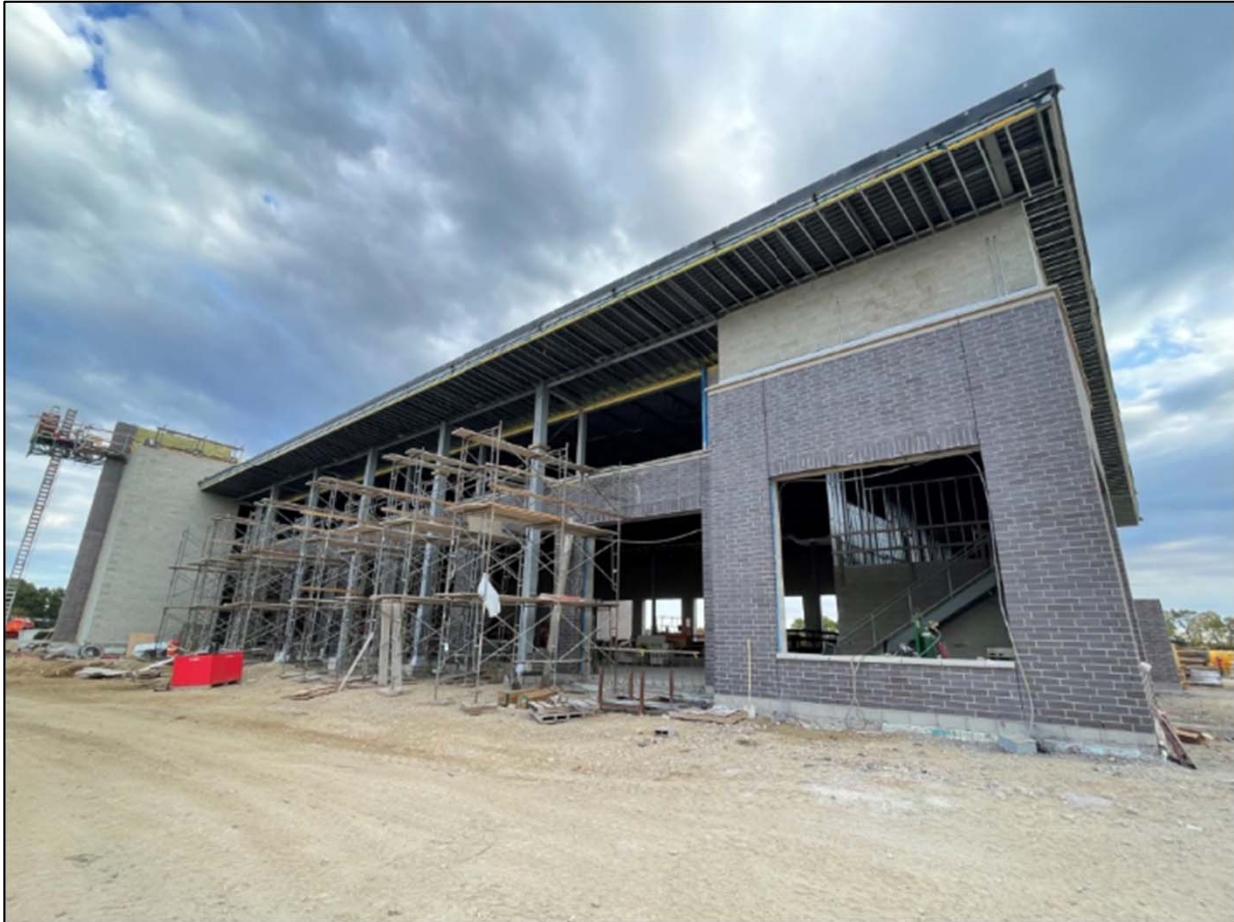
Masonry, Steel and Roof at Fire Department Apparatus Bays and Antique Bay
