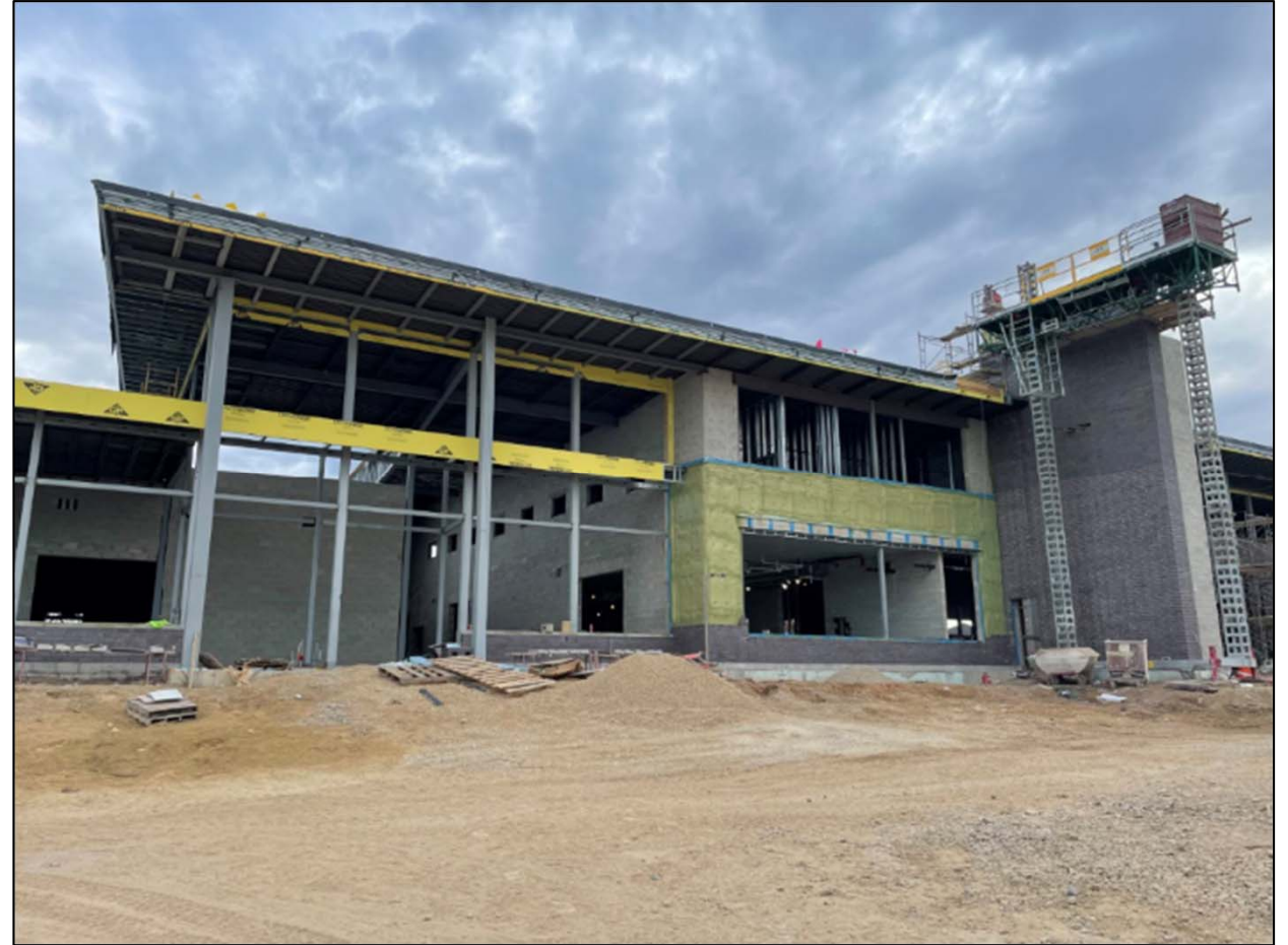
Masonry, Steel and Roofing work at Main Entry and Fire Department Staff Area
