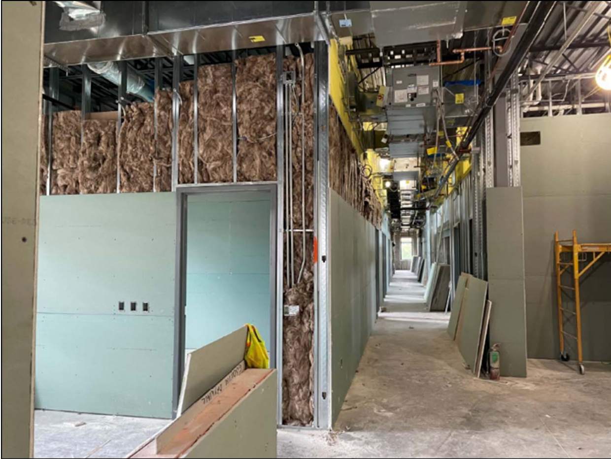
Drywall at Police Department Offices
