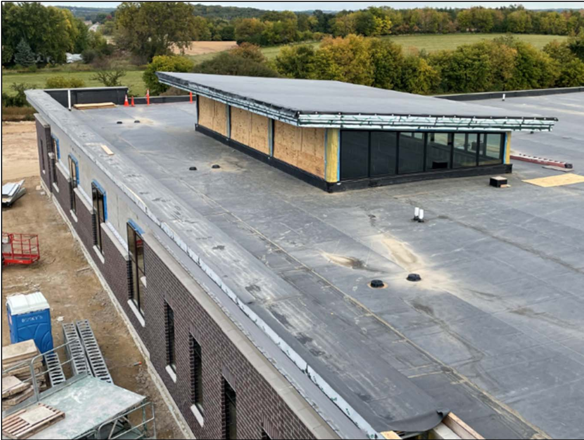
Clerestory at Squad Room
