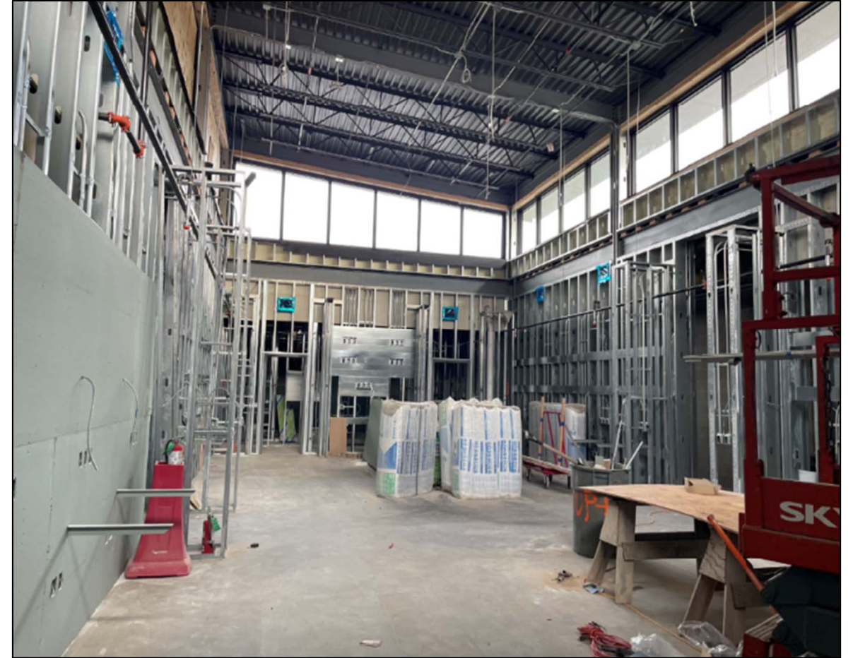
Blocking, Windows, Drywall at Squad Room
