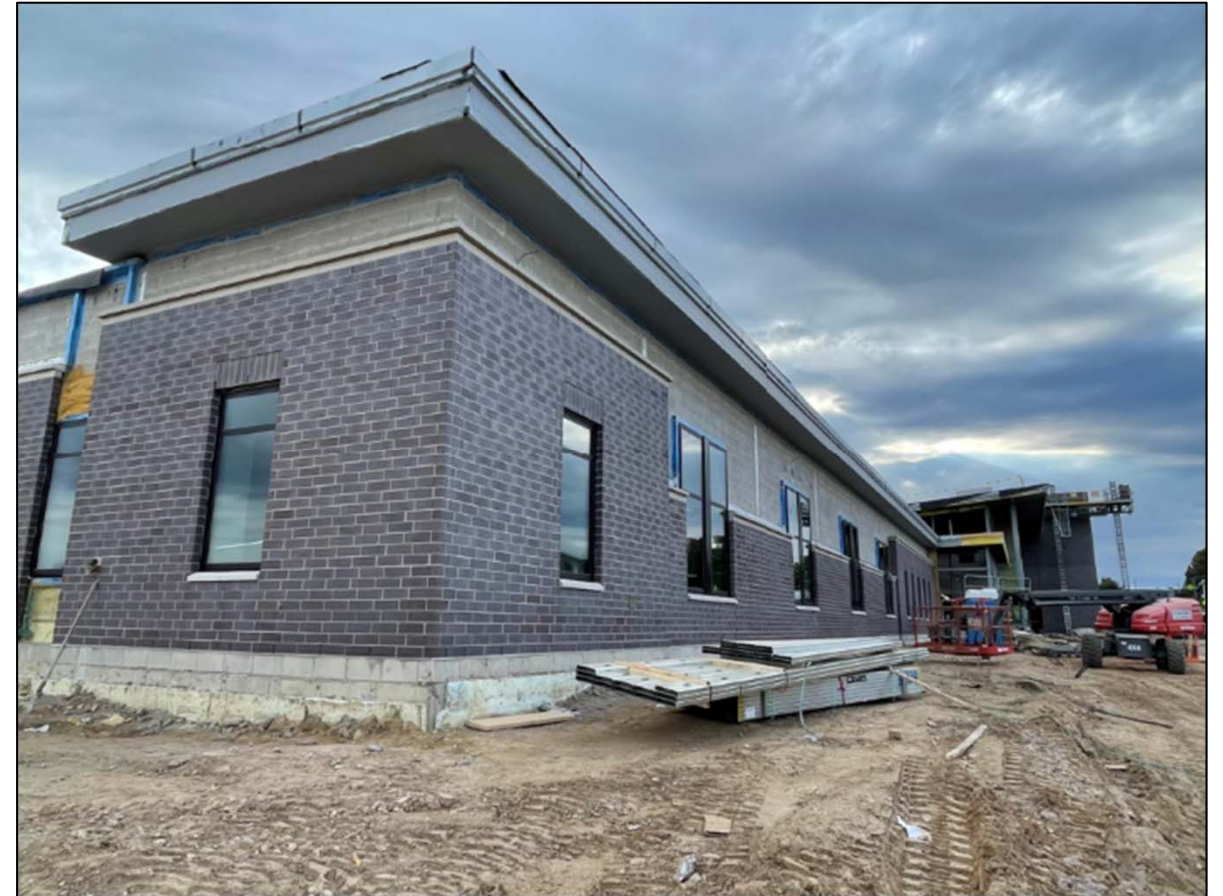
Brick, Windows, Roof at Police Department Offices
