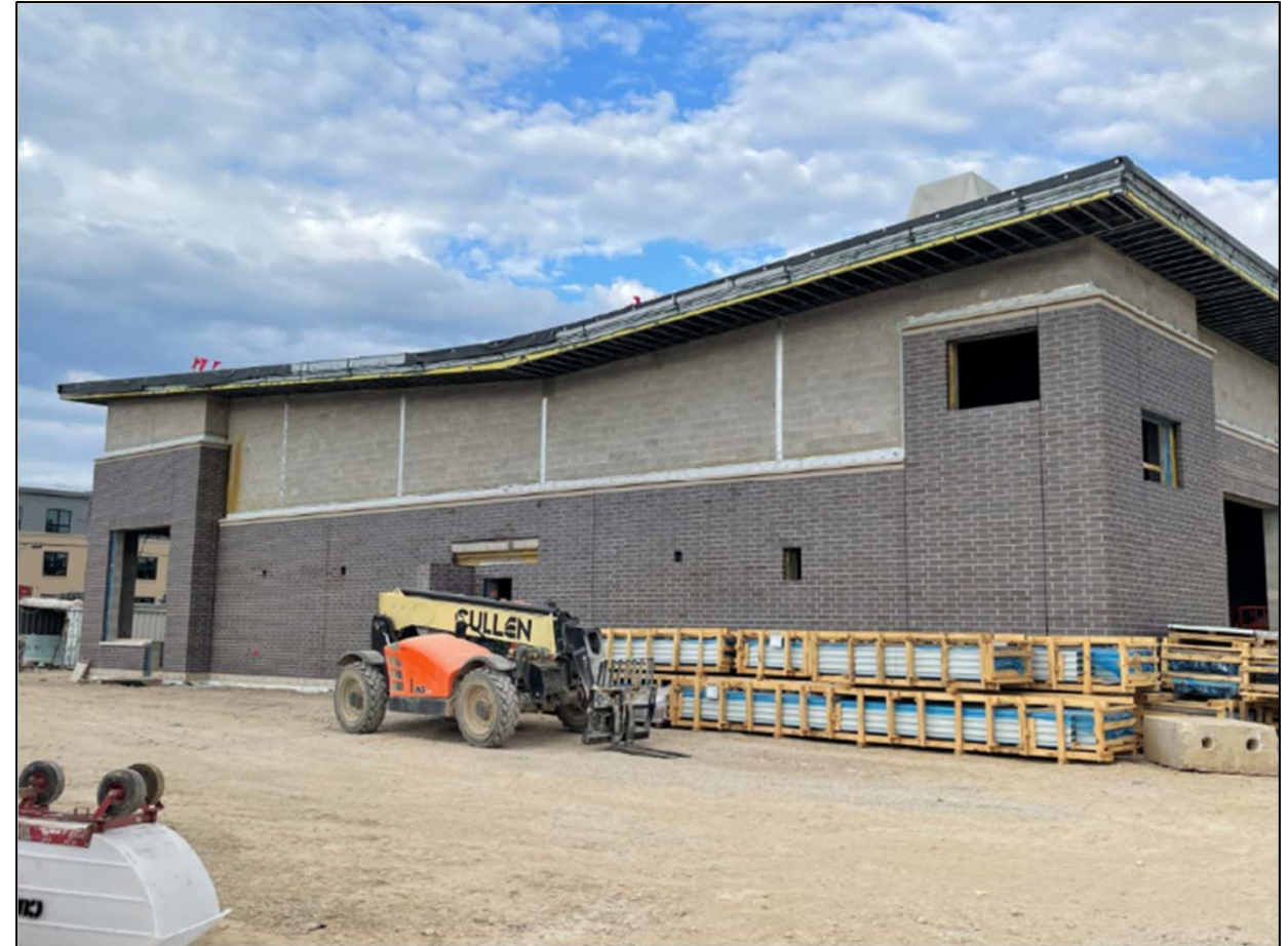
Fire Department West Elevation Ready for Metal Panel
