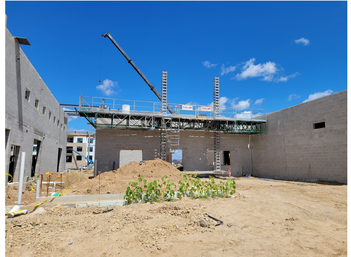
Construction of the last exterior wall is underway (courtroom)
