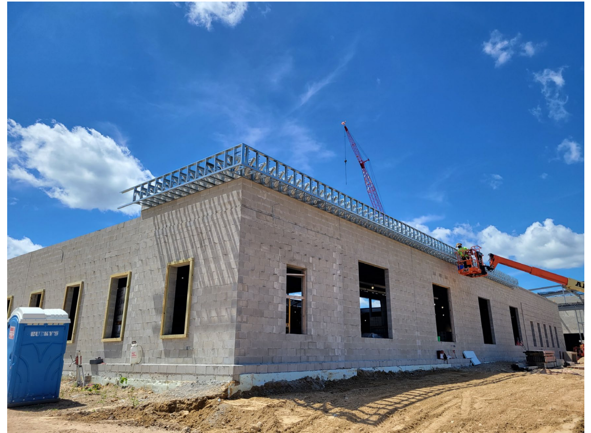
Exterior steel studs and wood blocking being completed
