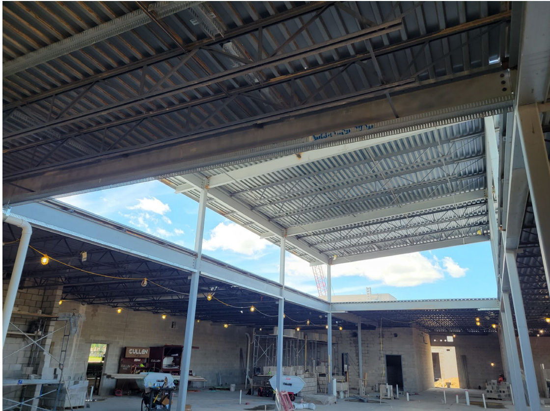
Structural Steel, joists and deck
