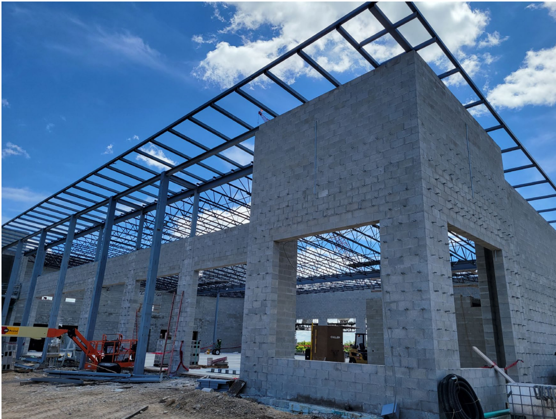
Structural steel and joists are in-place at the fire apparatus bay
