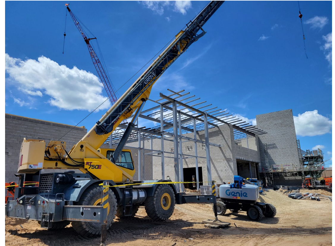
Structural steel has been erected at the main, secure entry
