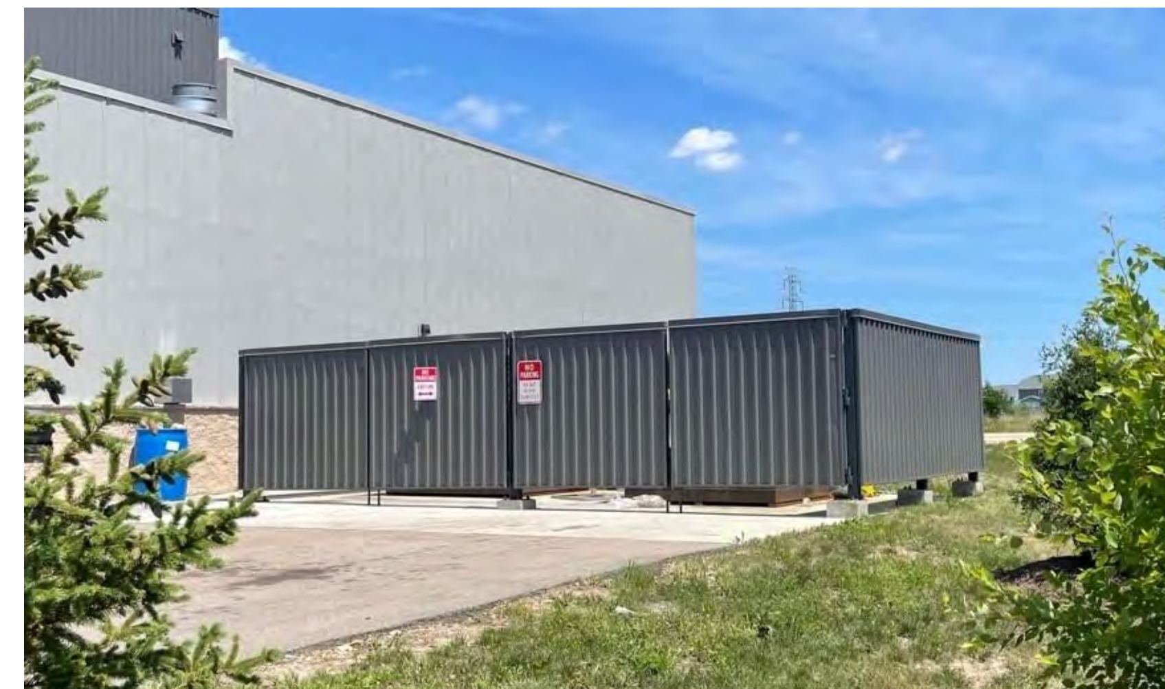
DUMPSTER ENCLSOURE- METAL FRAME AND PANEL
