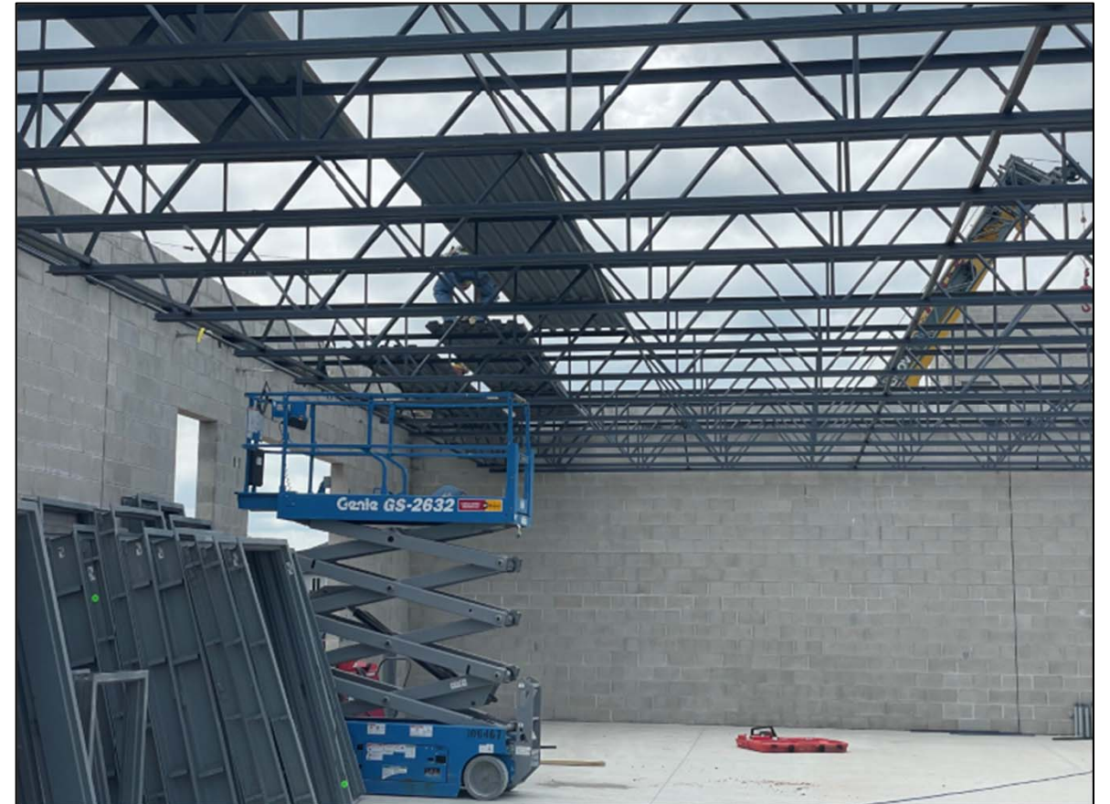
Police Garage Steel Deck Install and Hollow Metal Door Frames
