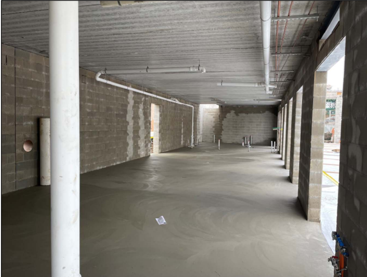
Fire Unit Turnout Gear Slab Poured
