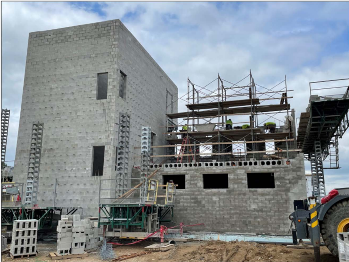
Hose Drying and Stair Tower (left) Exercise Room (right)
