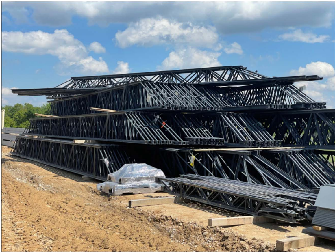
Much Anticipated Bar Joists ready for Install
