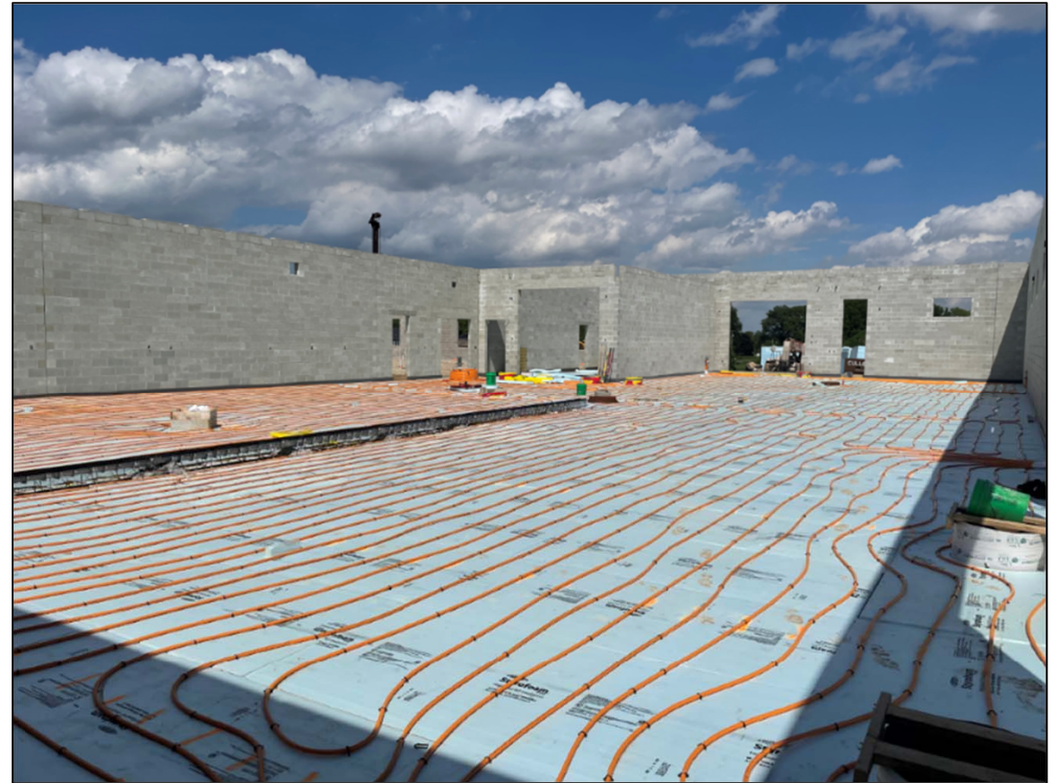
Completed Masonry Walls and Underslab Radiant Floor Piping at Police Garage and Sally Port
