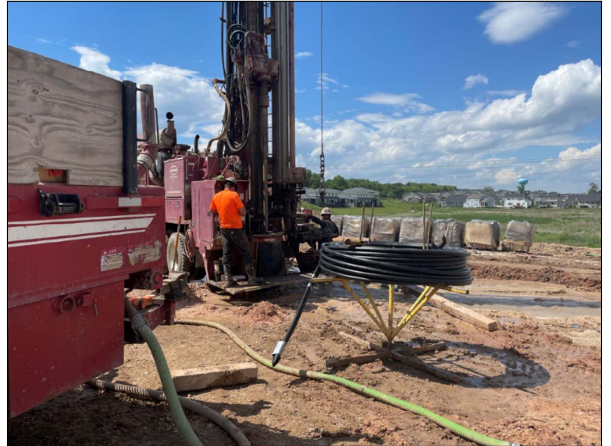
Geothermal Well Drilling
