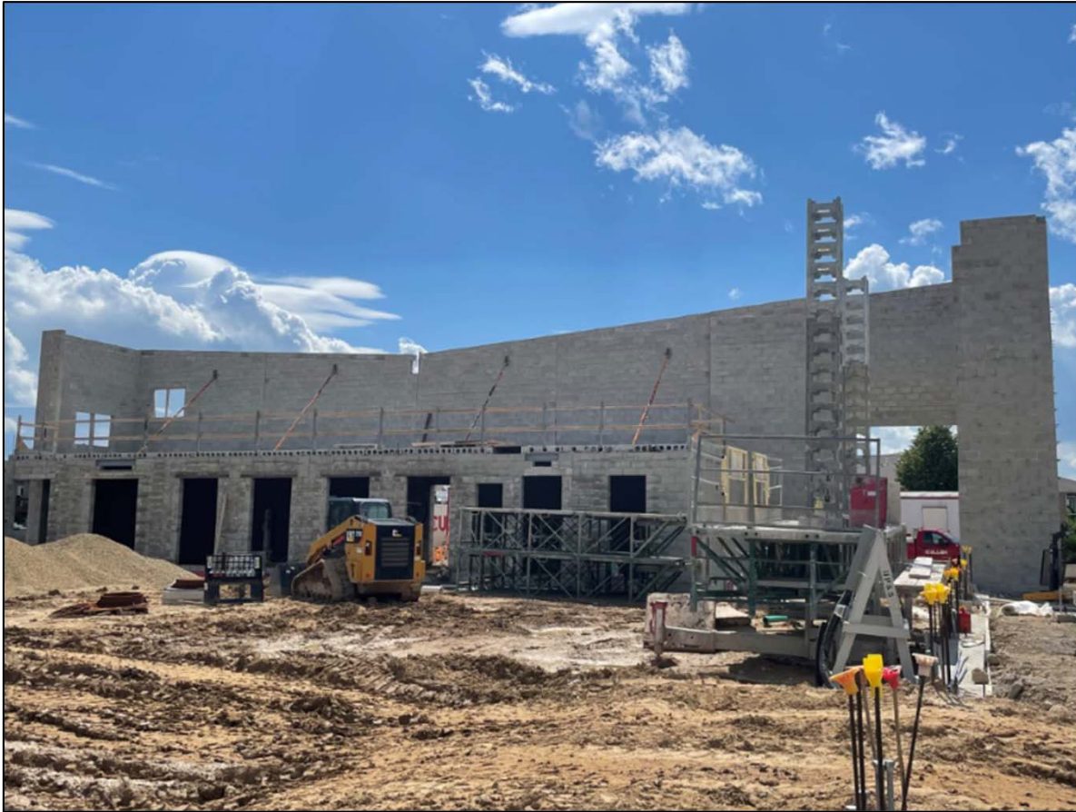
Fire Unit Mezzanine and Turnout Gear Masonry Is Up To Roof Level
