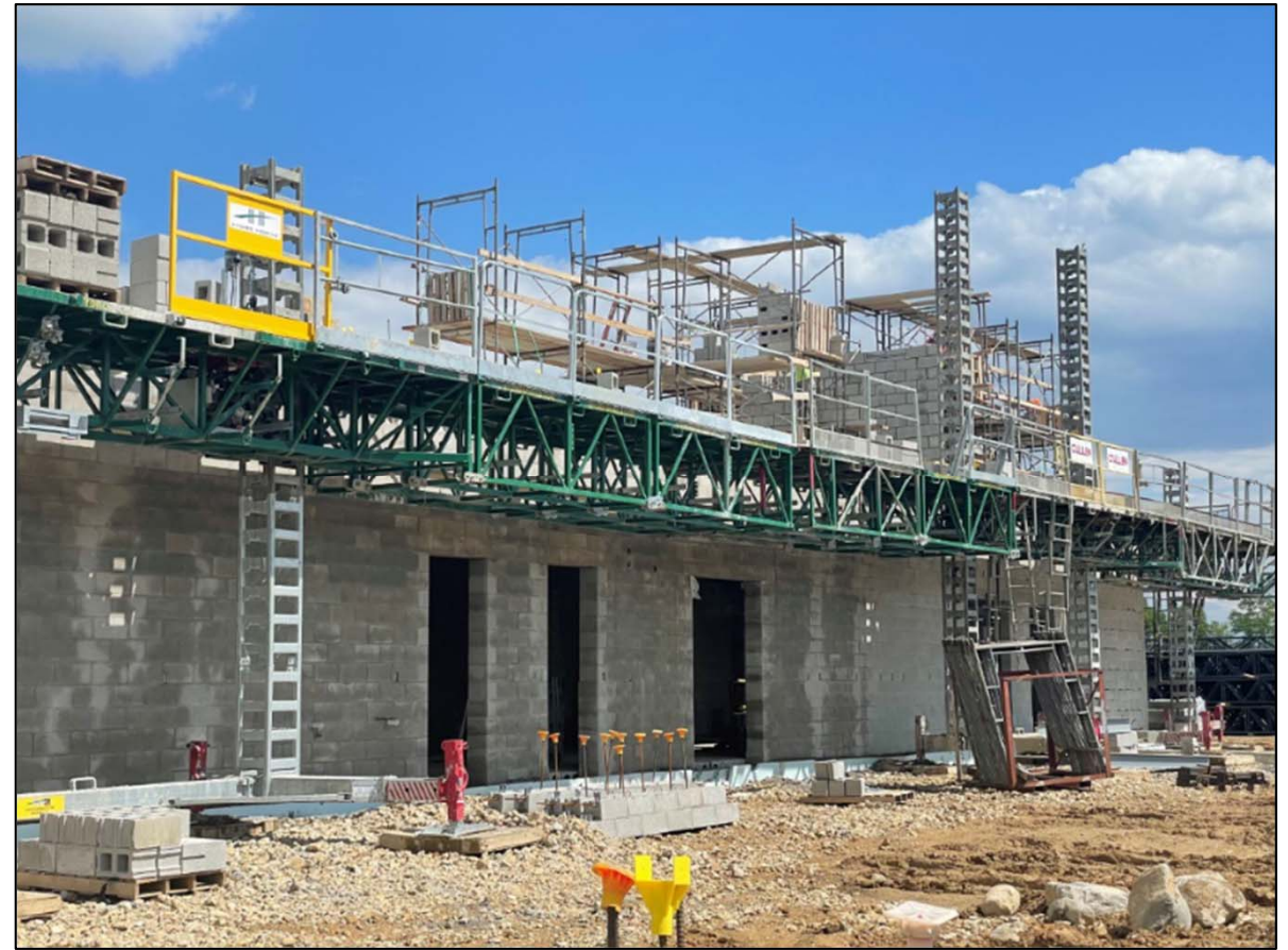
Lobby and Clerk Area Masonry Underway
