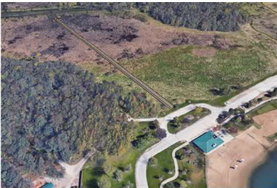
WETLAND BOARDWALK Located within close proximity to the Wruck Pavilion, a raised boardwalk provides the most direct route to Jerome Creek.
