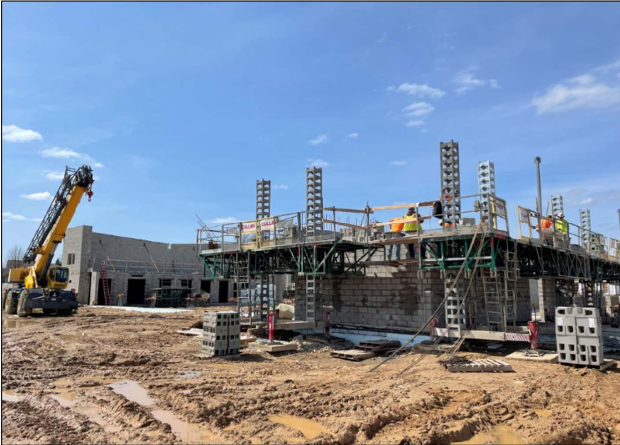
Masonry at Fire Unit Fitness Room (foreground) Fire Unit Mezzanine and Turnout Gear (background)
