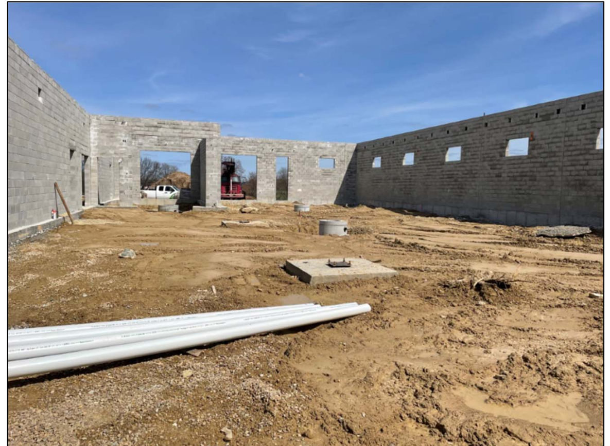
Masonry and Underslab Utilities at Police Garage and Sally Port
