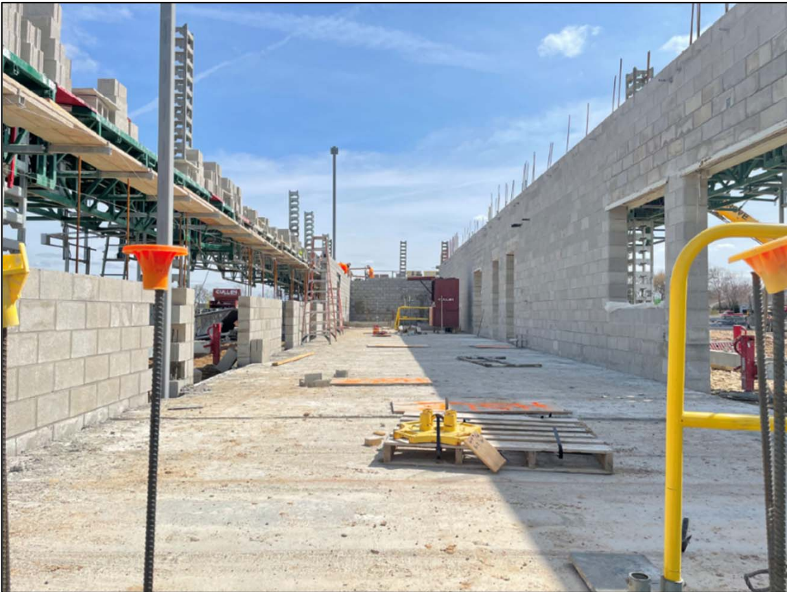
Precast Plank floor and Masonry Walls the the Fire Unit Mezzanine Level (Storage and Mechanical)
