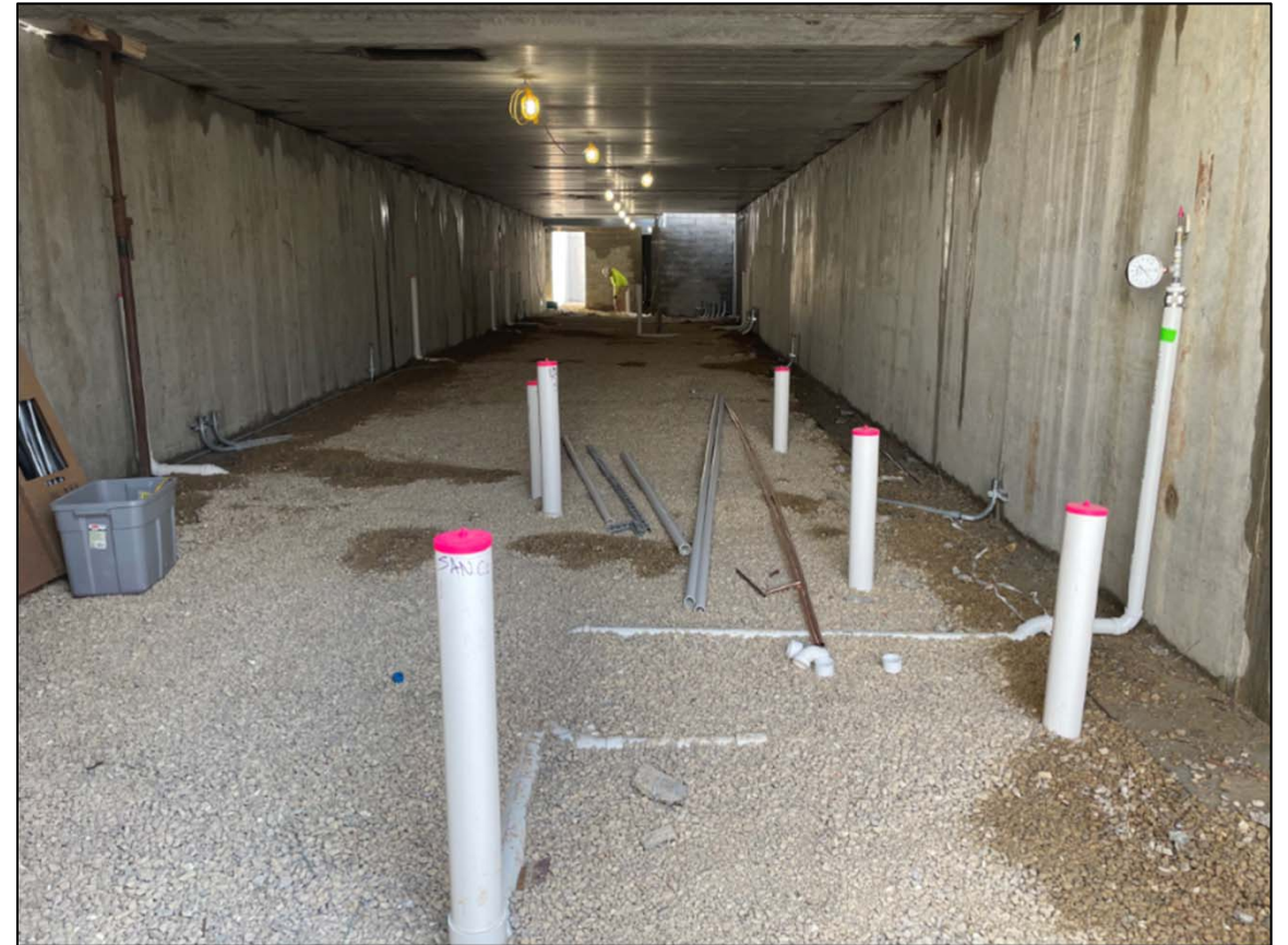
Underslab Utilities at Basement Level
