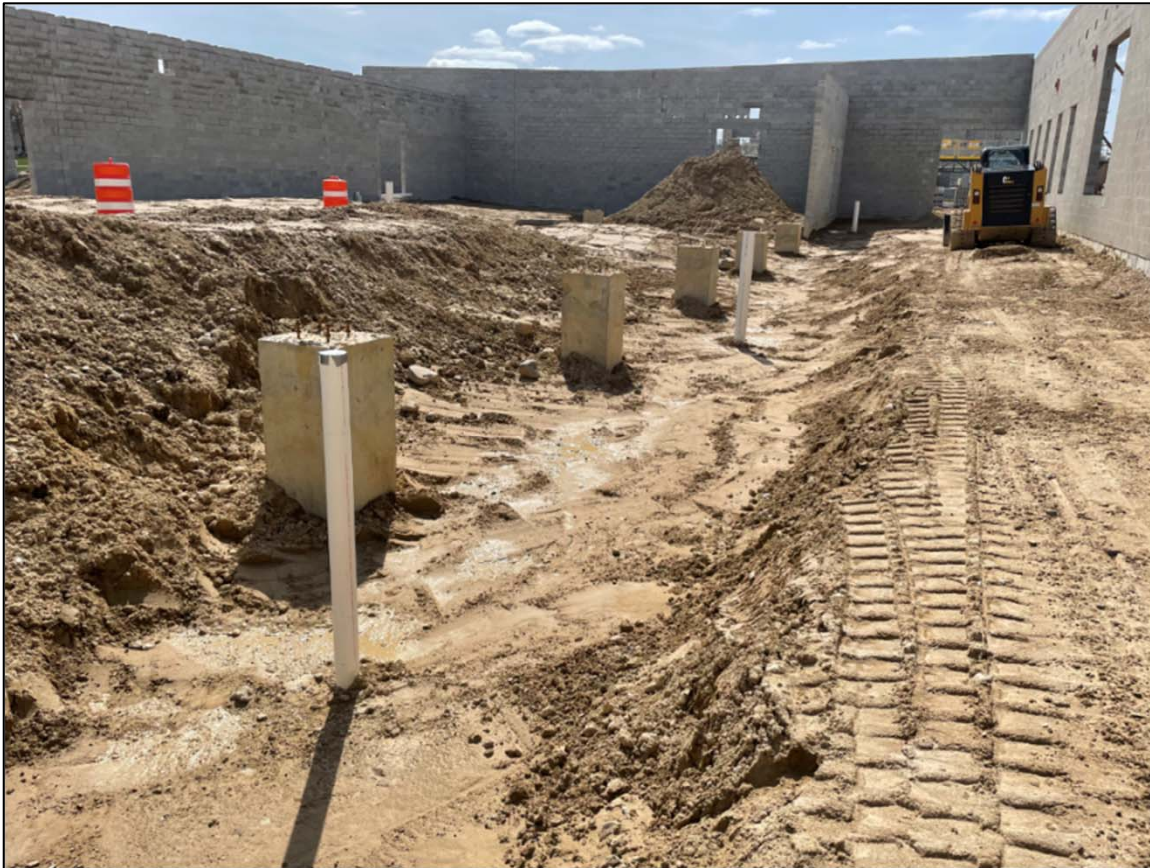
Underslab Utilities at Police Unit
