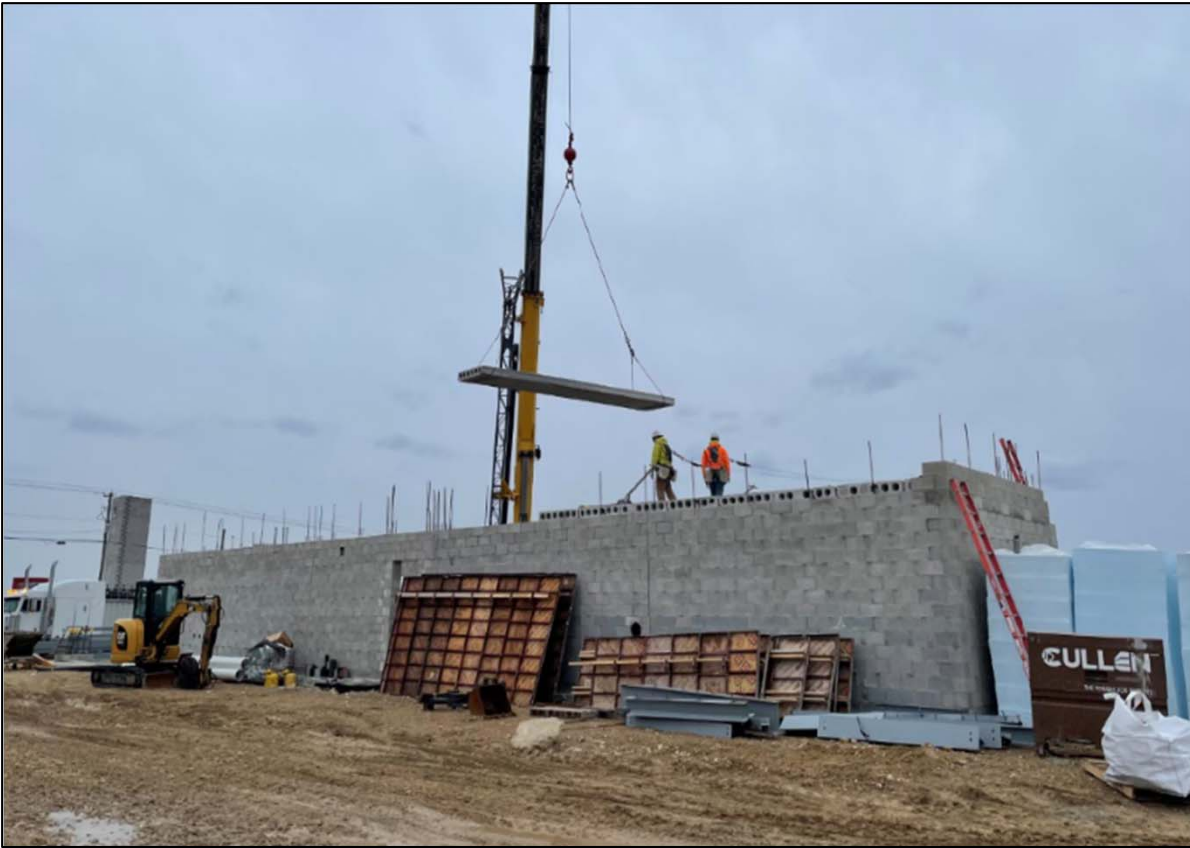
Precast Plank being set at Fire Unit Turn-Out Gear
