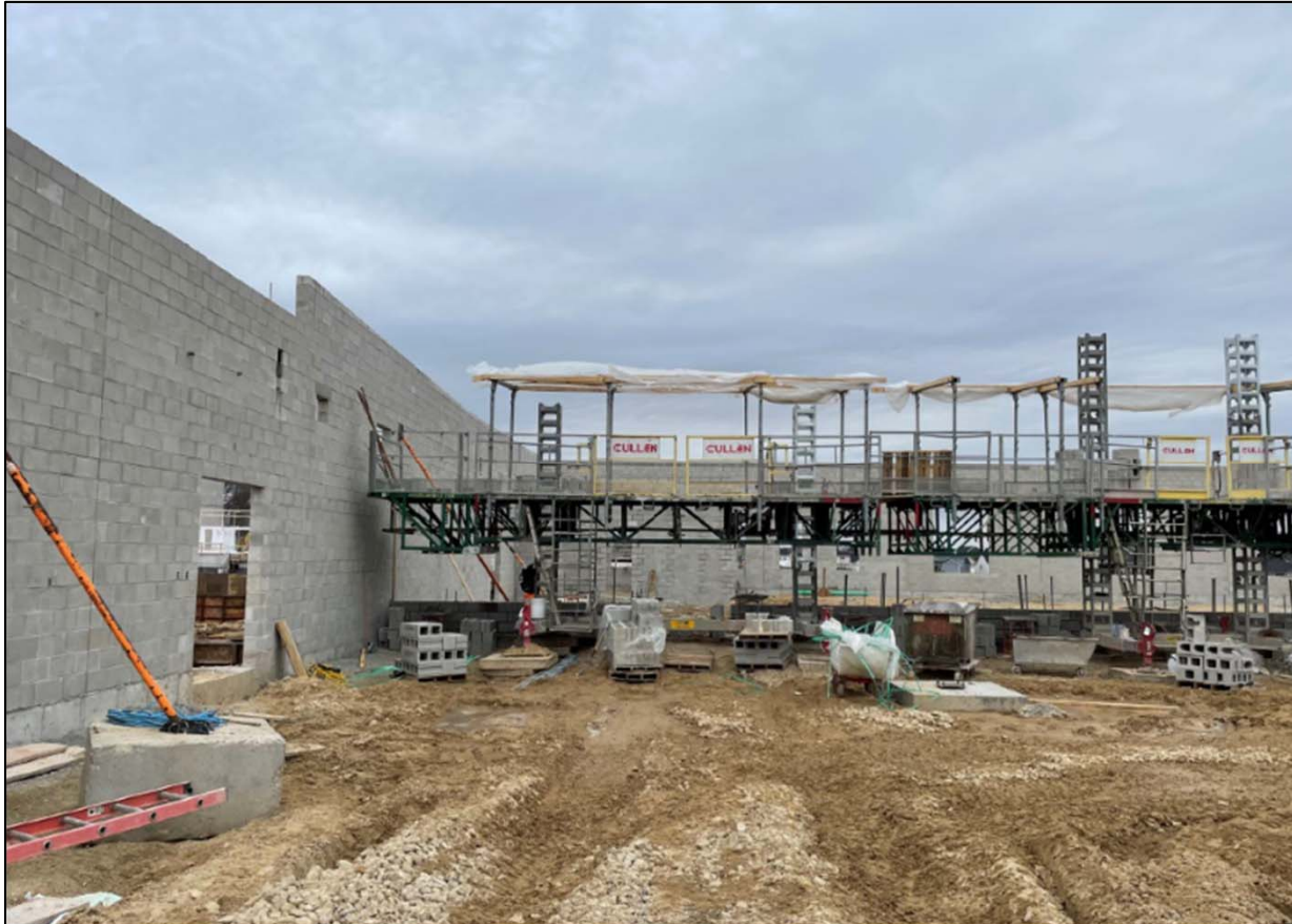
Masonry at Police Unit
