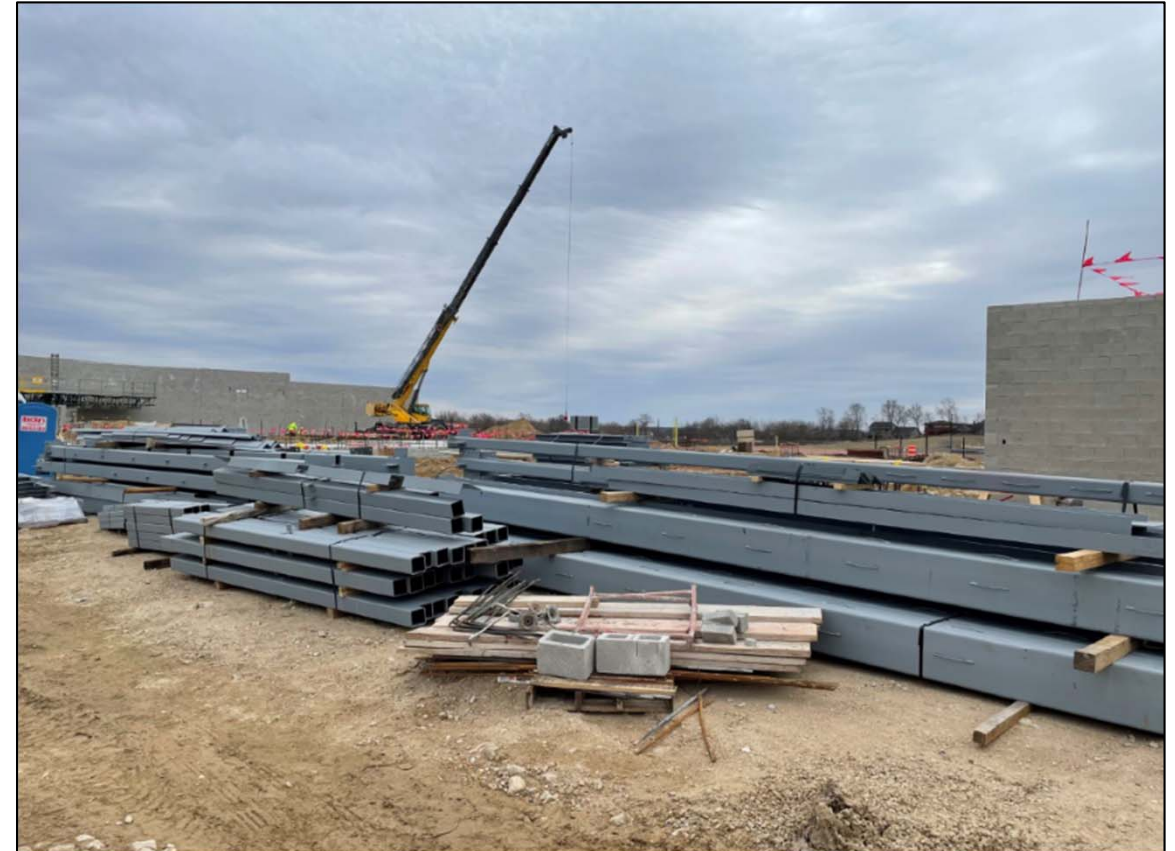
Structural Steel Received on Site
