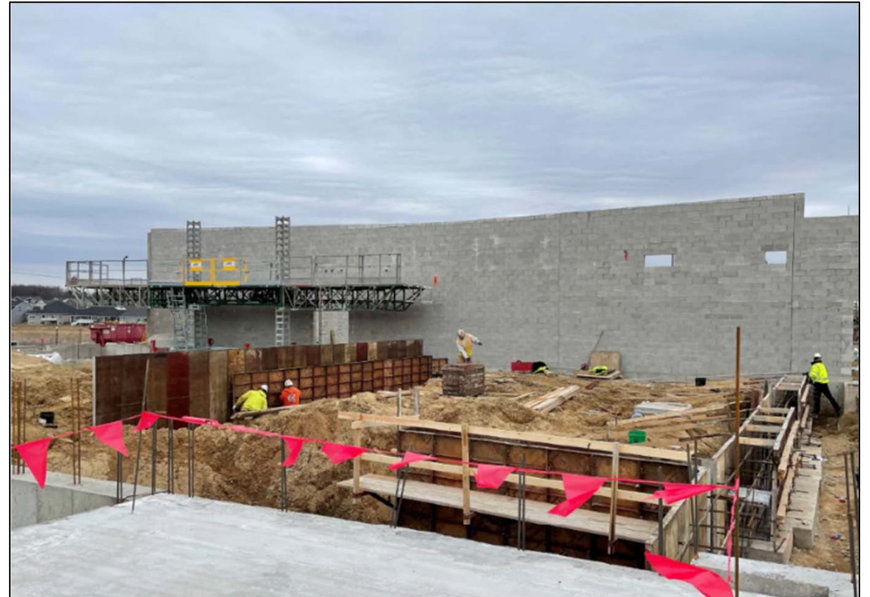
Footing Work at Interior Walls (Courts)
