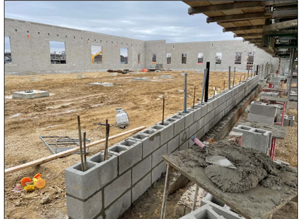
Interior Masonry wall at Police Unit/Garage
