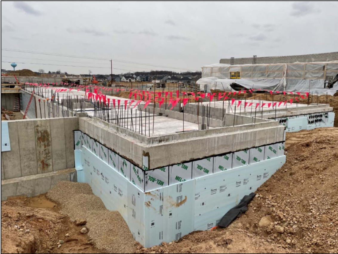
Basement Foundation Walls with Precast Plank (foreground) Masonry HydroMobile setup (background is PD)
