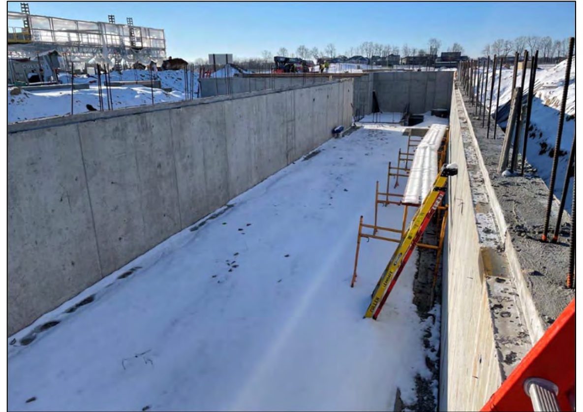
Foundation work at Basement and Elevator
