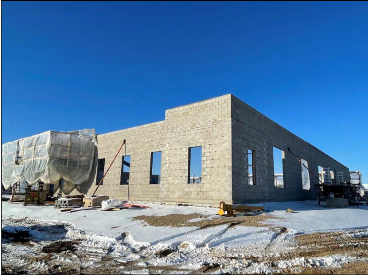
Masonry at Police Unit
