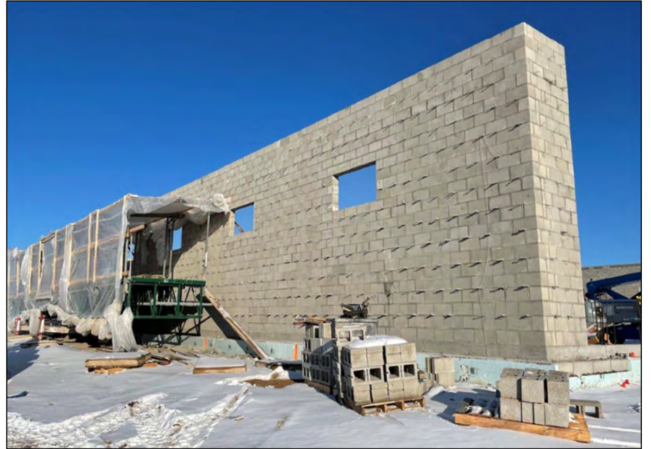
Masonry at Police Garage
