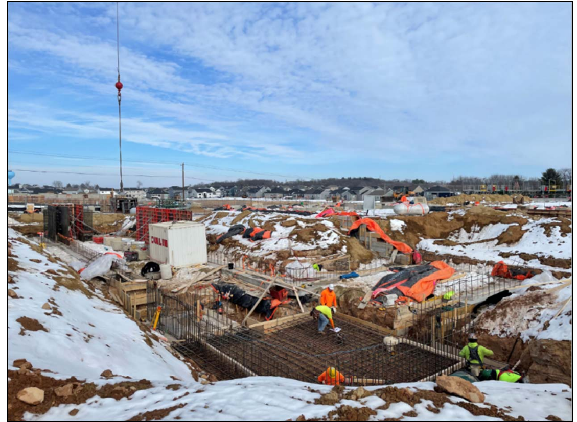
Foundation work at Basement and Elevator
