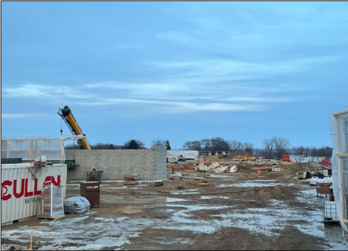
Fire Unit Masonry Walls (foreground) Police Unit Masonry Walls (background)
