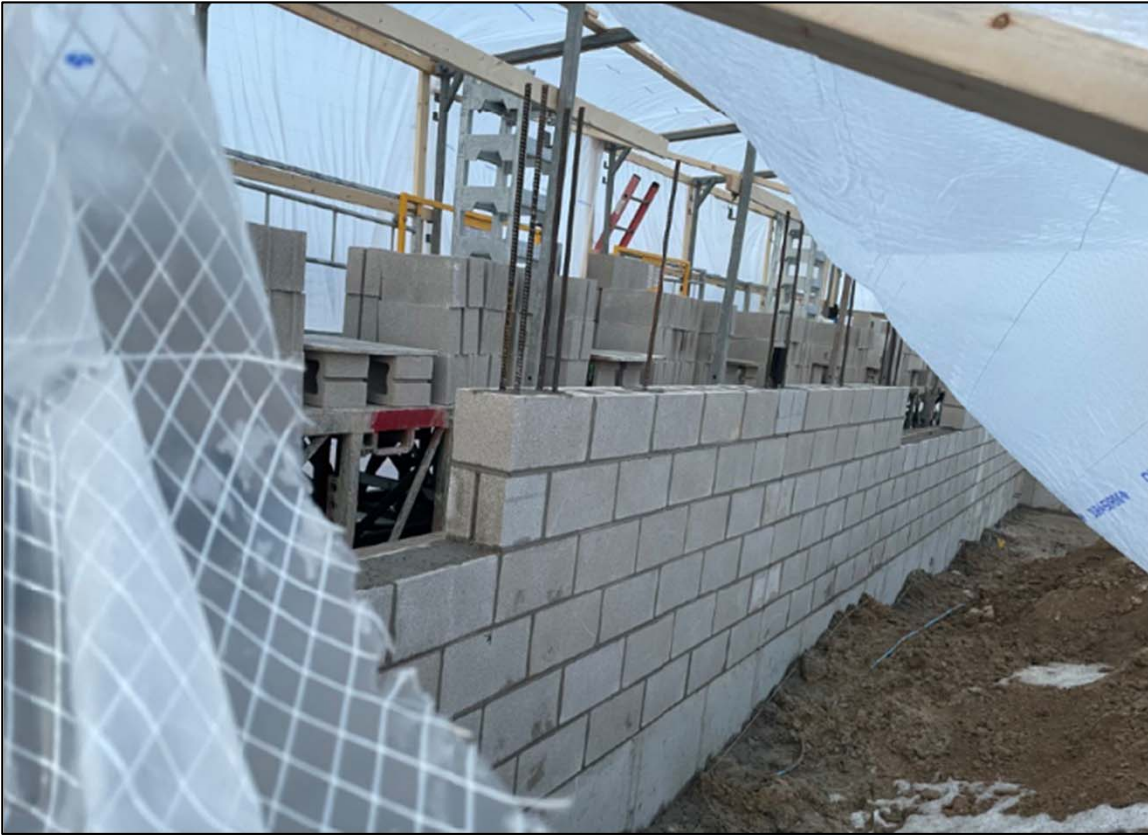
Masonry at Police Unit
