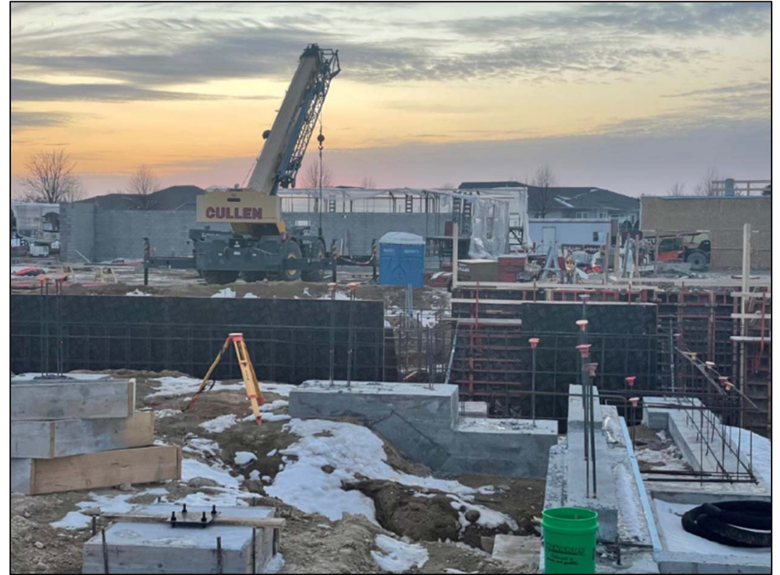
Basement Foundation Walls (foreground) Masonry Walls (background)
