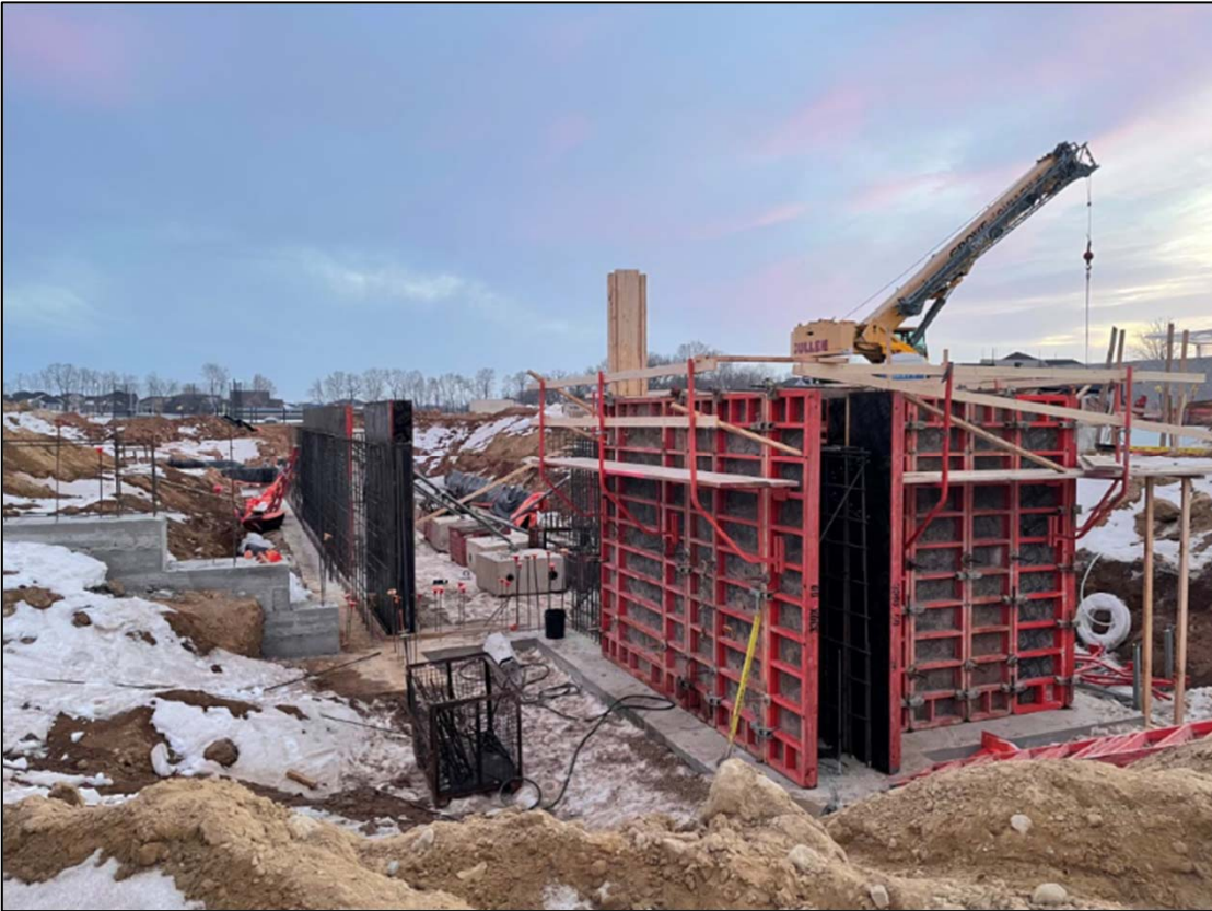
Basement Foundation Walls
