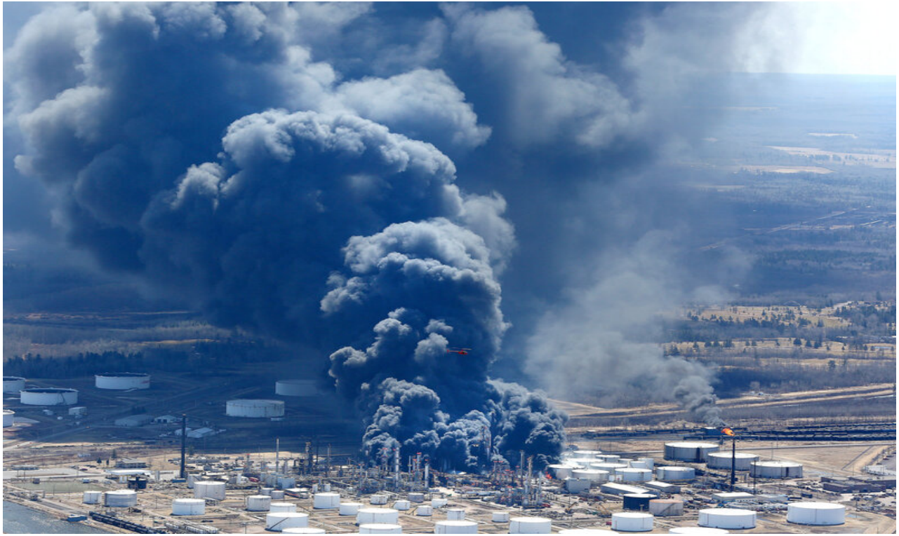
Figure 1 April 2018 Husky Tank Farm Explosion (Superior, WI) caused by faulty valve.
