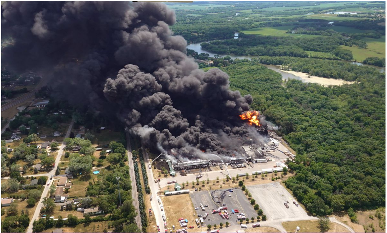
Figure 2 June 2021 Rockton, IL Plant Explosion caused by human error.
