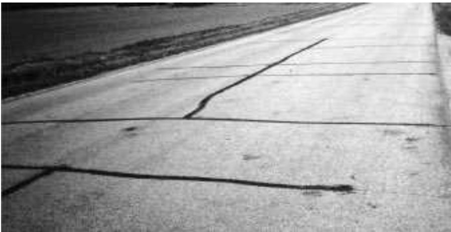
▼ Open crack, 1/2" wide; adjoining pavement sound.
