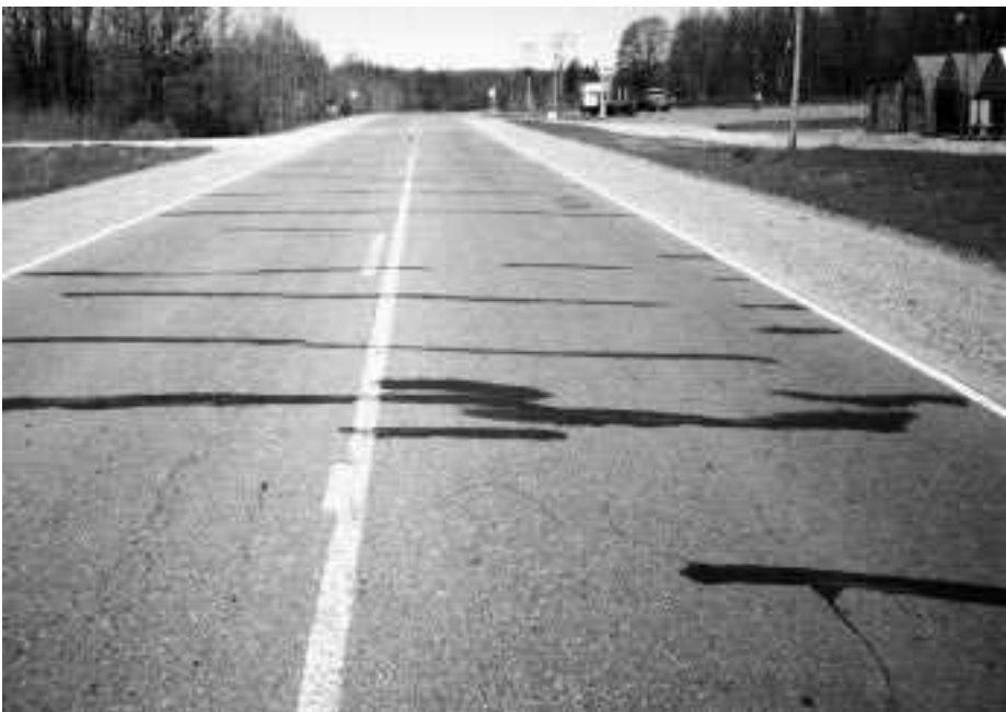
◀ Sealed cracks, a few feet apart.
