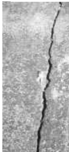
▼ Open crack, 1/2" wide; adjoining pavement sound.
