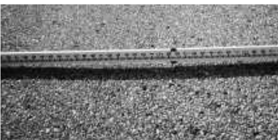
▼ Extensive block cracking. Blocks tight and sound. ◀ Slight rutting in wheel path.
