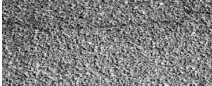
◀ Slight raveling. Small aggregate particles have worn away exposing tops of large aggregate.
