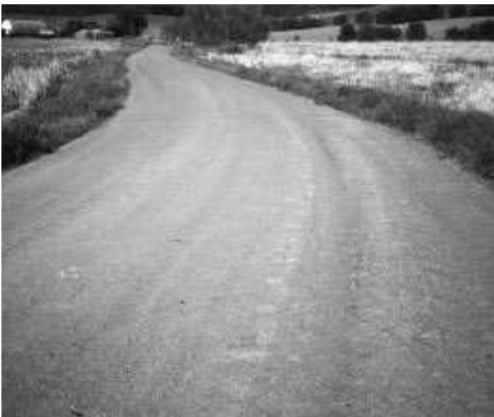
▲ New cold mix surface.
