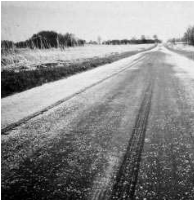
▼ Severe flushing.
