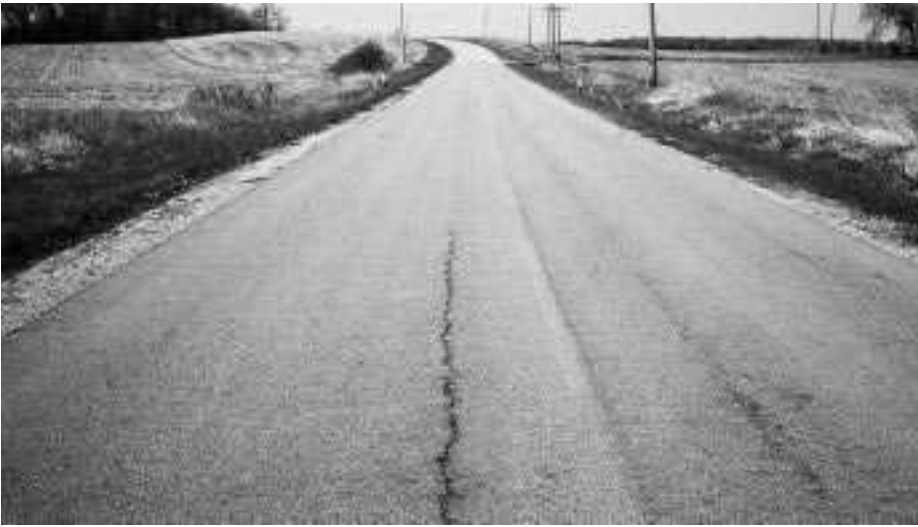
▼ Slight rutting; patch in good condition.
