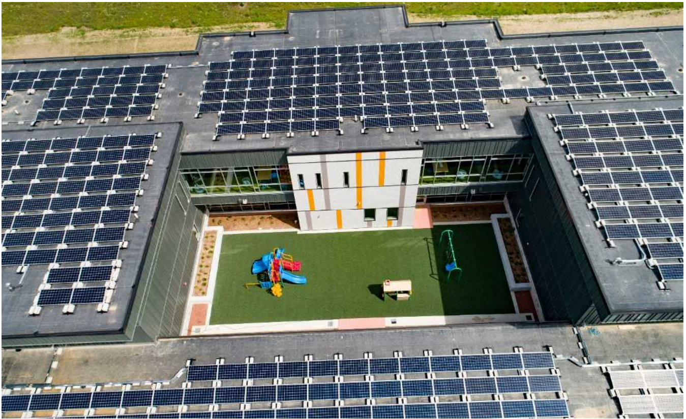
Figure 6- Closer image of solar PV panel and racking arrangement - similar design assumptions have been made for the new PSB project
