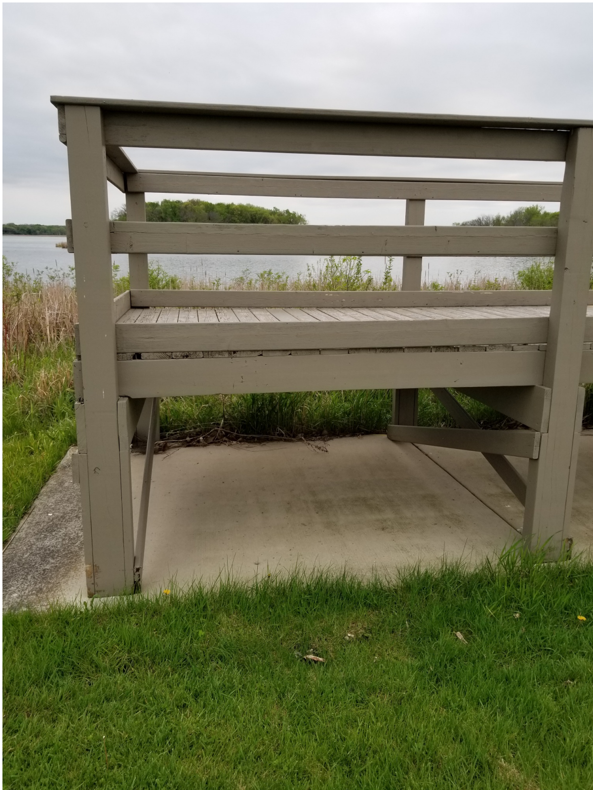
Boardwalk install location
