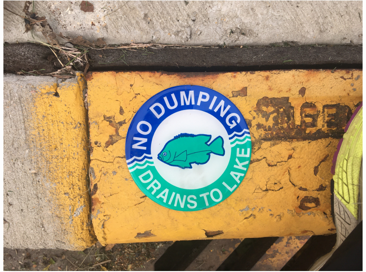
Storm Drain with new Decal, rated to last 10-12 years
