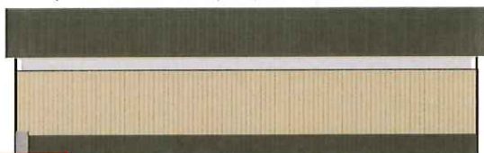
North Side Wall 1 on Building 1
