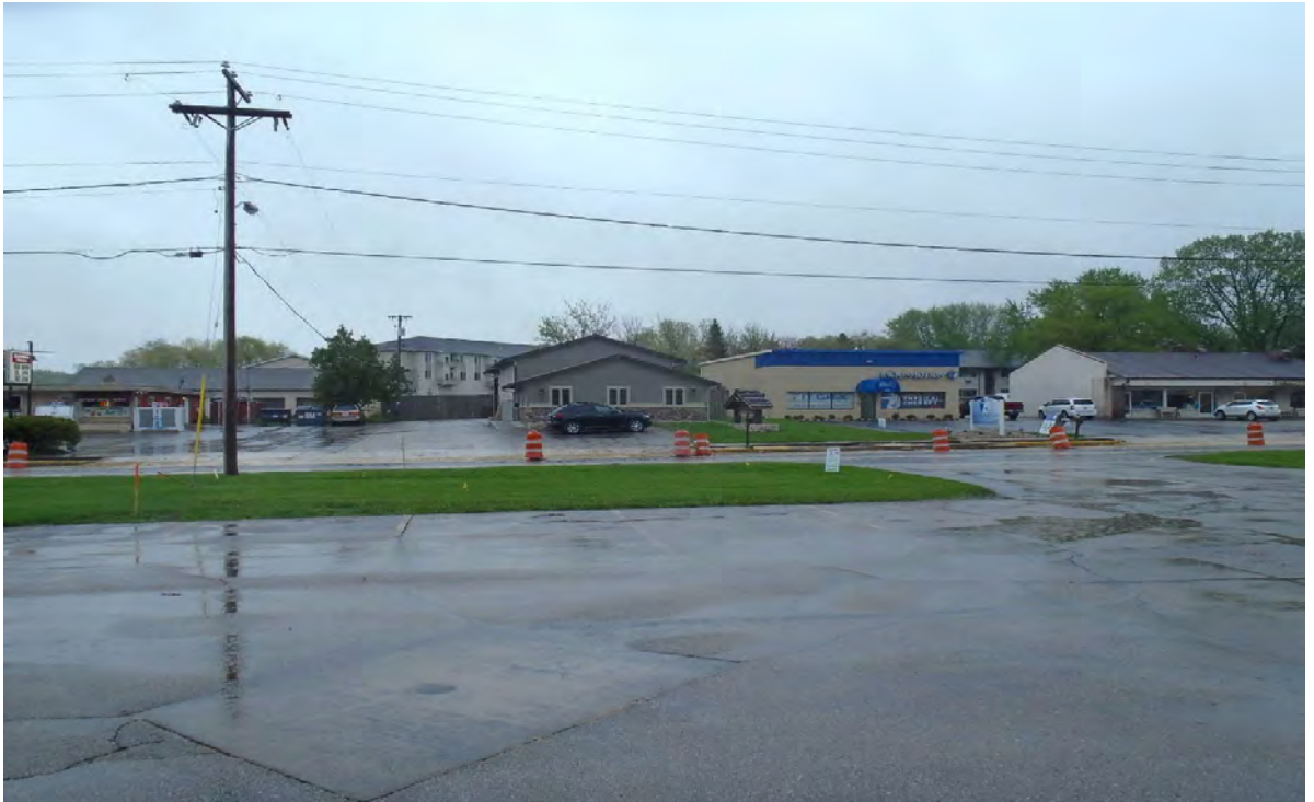
Photo 7 – Commercial buildings north of 4719 Farwell St, including the 4720 Farwell LUST property.
