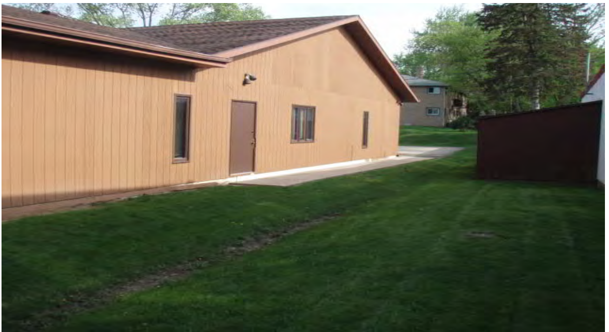
Photo 8 – West wall and west property line of commercial building at 4719 Farwell St and the adjacent Ken's Automotive Service building in photo right.
