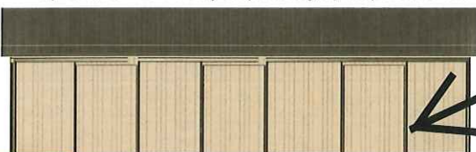
South Side Wall 2 on Building 1
