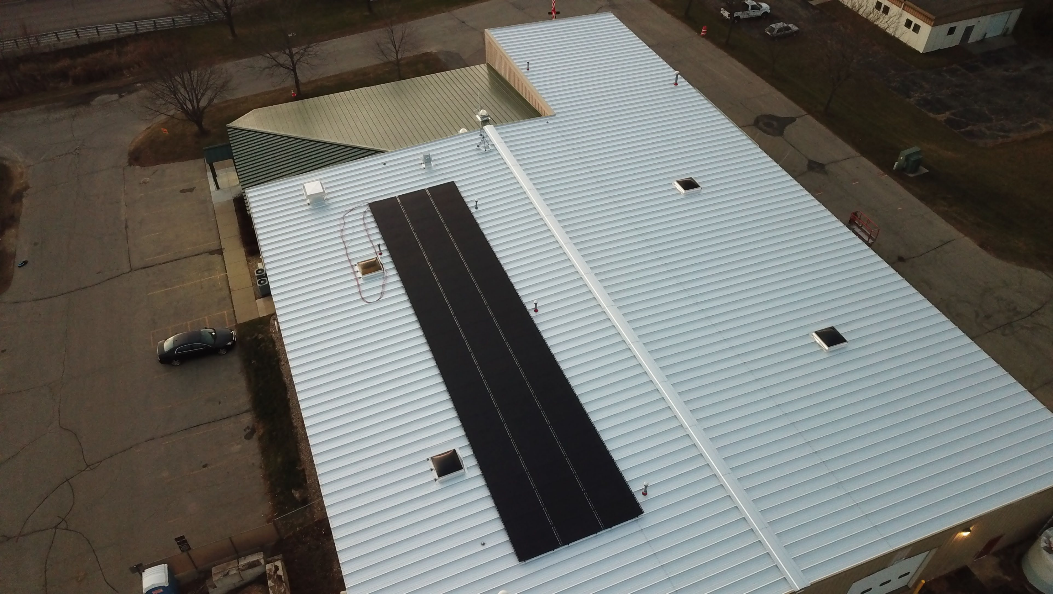
Public Works Building – Rooftop Solar, 23 kW DC solar PV array (2021)
